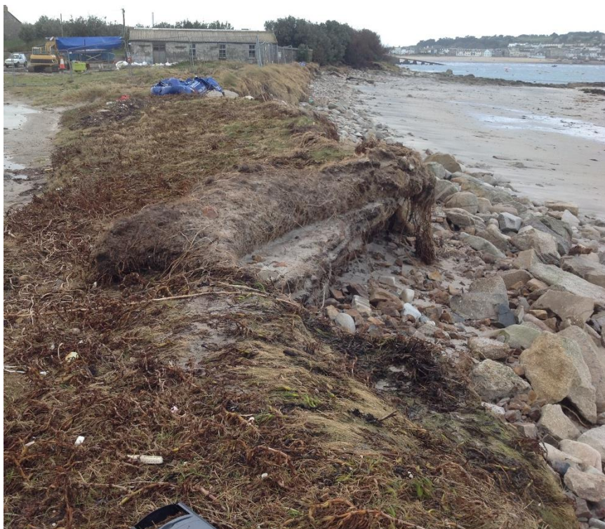
Erosion of Porthloo bank following 2014 storms (photo courtesy of Duchy of Cornwall)
