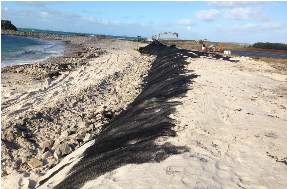
Works repairing the bank at Periglis following the 2014 storms (photo courtesy of the Duchy of Cornwall)
