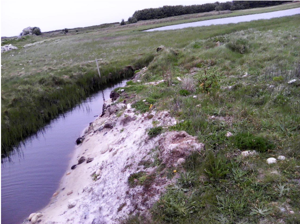
The Leat at Big Pool, St Agnes developed to release sea water from the area after flood events
