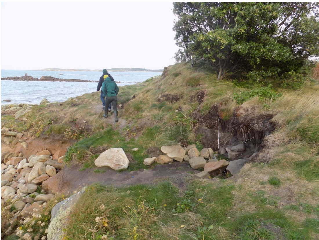
Fig 5 November 2016: an area of coastal erosion affects a small section on the southern low cliff face of the promontory.
