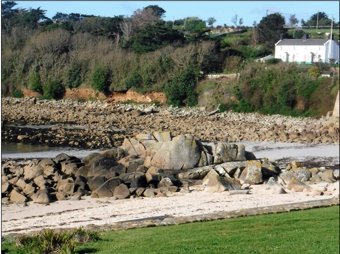
Fig 16 Erosion below the Garrison Walls near Little Porth, 29 April 2018 (photo: CAU).
