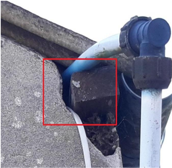
Photo 8. Gap behind wall plate for services
