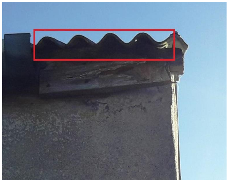
Photo 11. Gaps between wall plate and corrugated roof sheets
