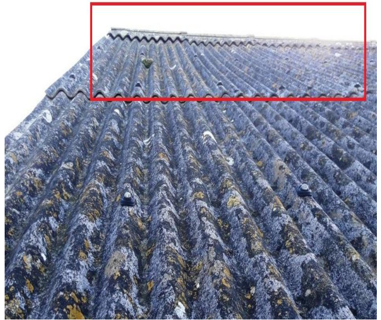
Photo 9. Gap between roof ridge tile and corrugated roof sheet
