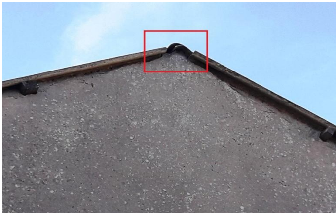
Photo 2. Gap between wall plate and block work
