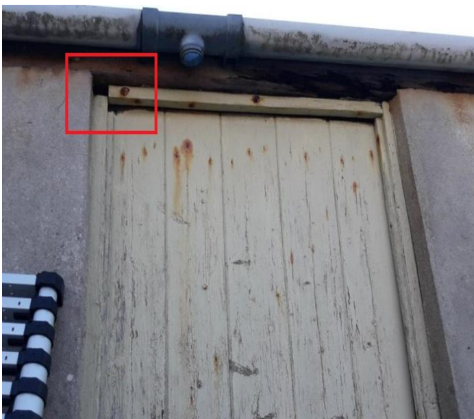
Photo 10. Gap in wooden surround of 1 st floor hatch
