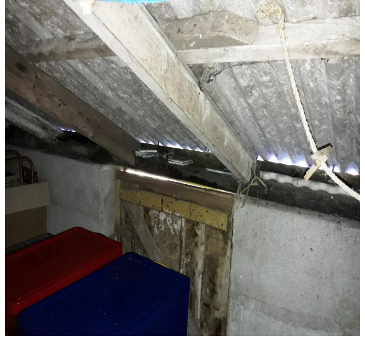
Photo 13. 1 st floor showing exposed roof sheets
