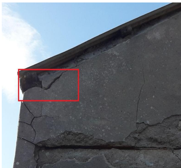
Photo 6. Crack in render and gap behind wall plate
