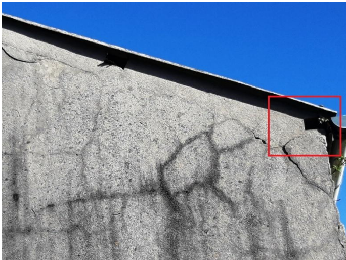
Photo 2. Gap between wall plate and block work
