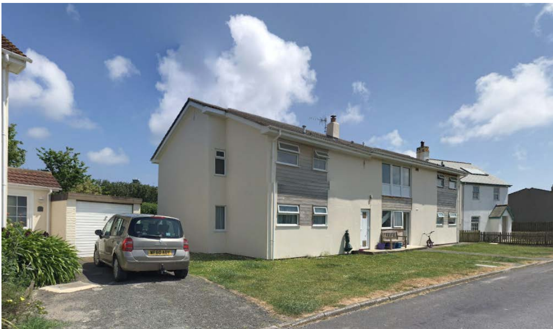
FIGURE 6 COUNCIL HOUSING, ENNOR CLOSE, ST MARY'S
