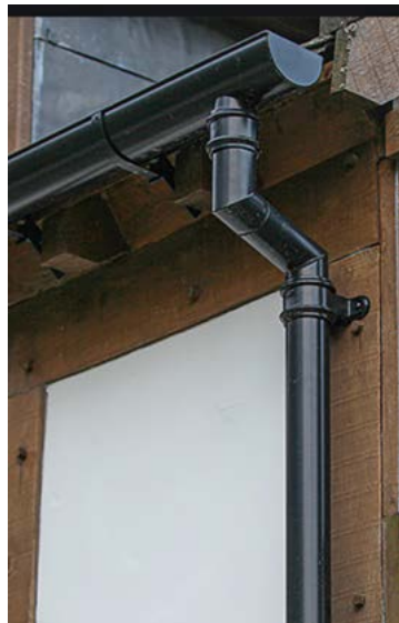
Swan neck gutter on rafter brackets
