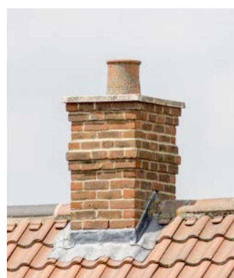
Brickwork chimney stack
