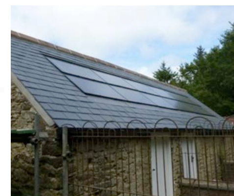
In roof PV's or solar slates at rear
