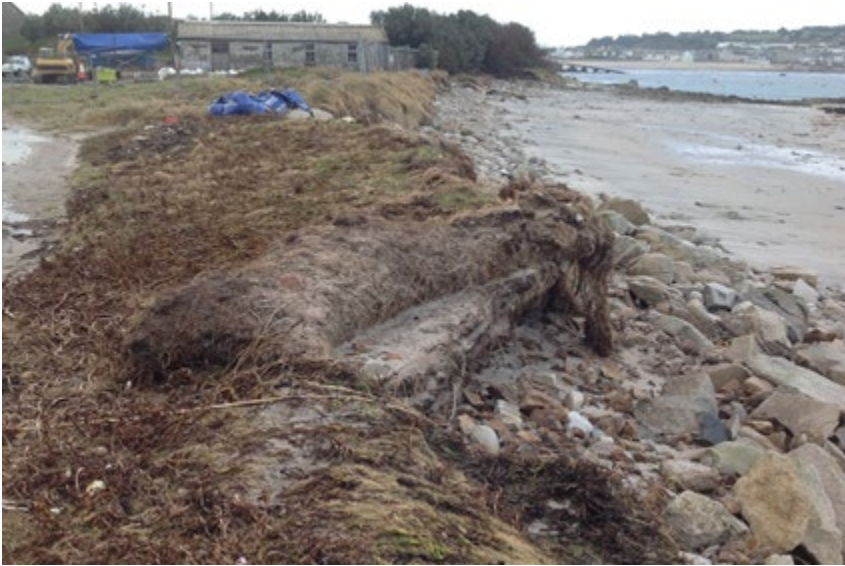
Porthloo, St Mary's Erosion of Porthloo bank following 2014 storms (photo courtesy of Duchy of Cornwall)
