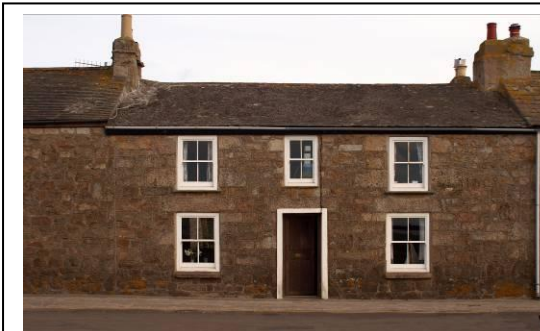
Combined granite rubble and dressed granite stacks, the Strand, St Mary's
