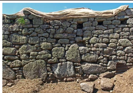
Tean Farmhouse ruin, Tean (rear wall joist-socket evidence for former loft within roof space)
