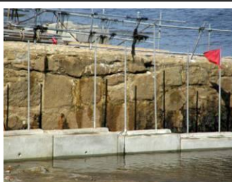
St Agnes, C19 quay walls during 2007 works that encapsulated the old walls
