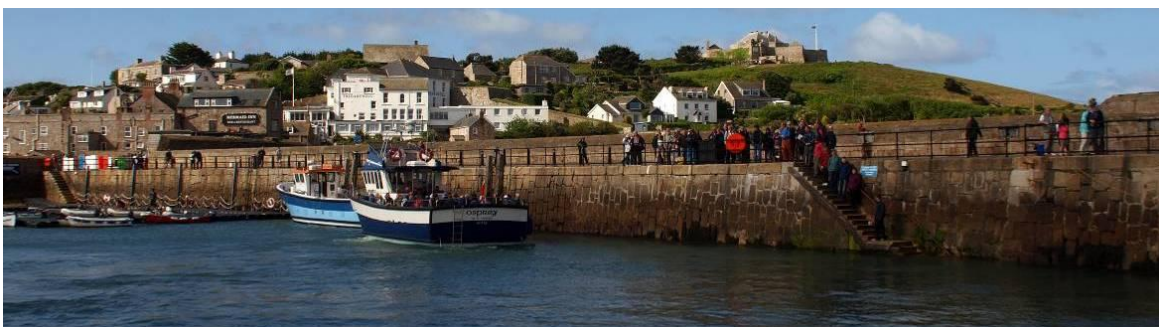
ST. MARY'S, HUGH TOWN: The Pier ( II) Quay and breakwater, begun by Francis Godolphin soon after 1601, rebuilt 1740 and 1748; new pier extending north to Rat Island built 1835-8 for Augustus Smith, Lord Proprietor of the Islands; lengthened 1889 for the flower trade; the construction of a pier for the new harbour, St. Mary's Port, was associated with the fortification of the Hugh begun by Godolphin which included Star Castle and the Garrison walls (q.v.) (from list description)
