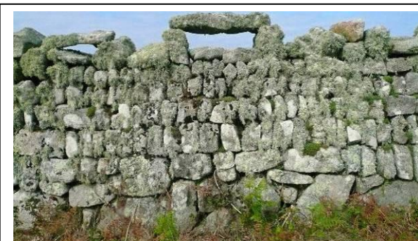
Samson, Deer Park walls: Built for Augustus Smith in circa the 1850's (rubble stone with sea-shell infill)
