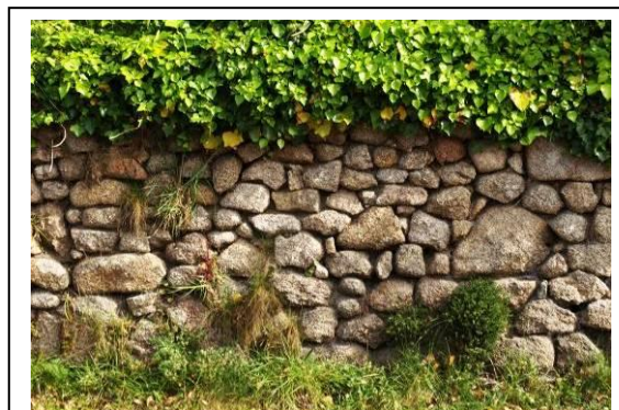
St Mary's: Old granite rubble retaining wall
