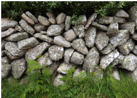
St Martin's: Field boundary (single-stone thickness)
