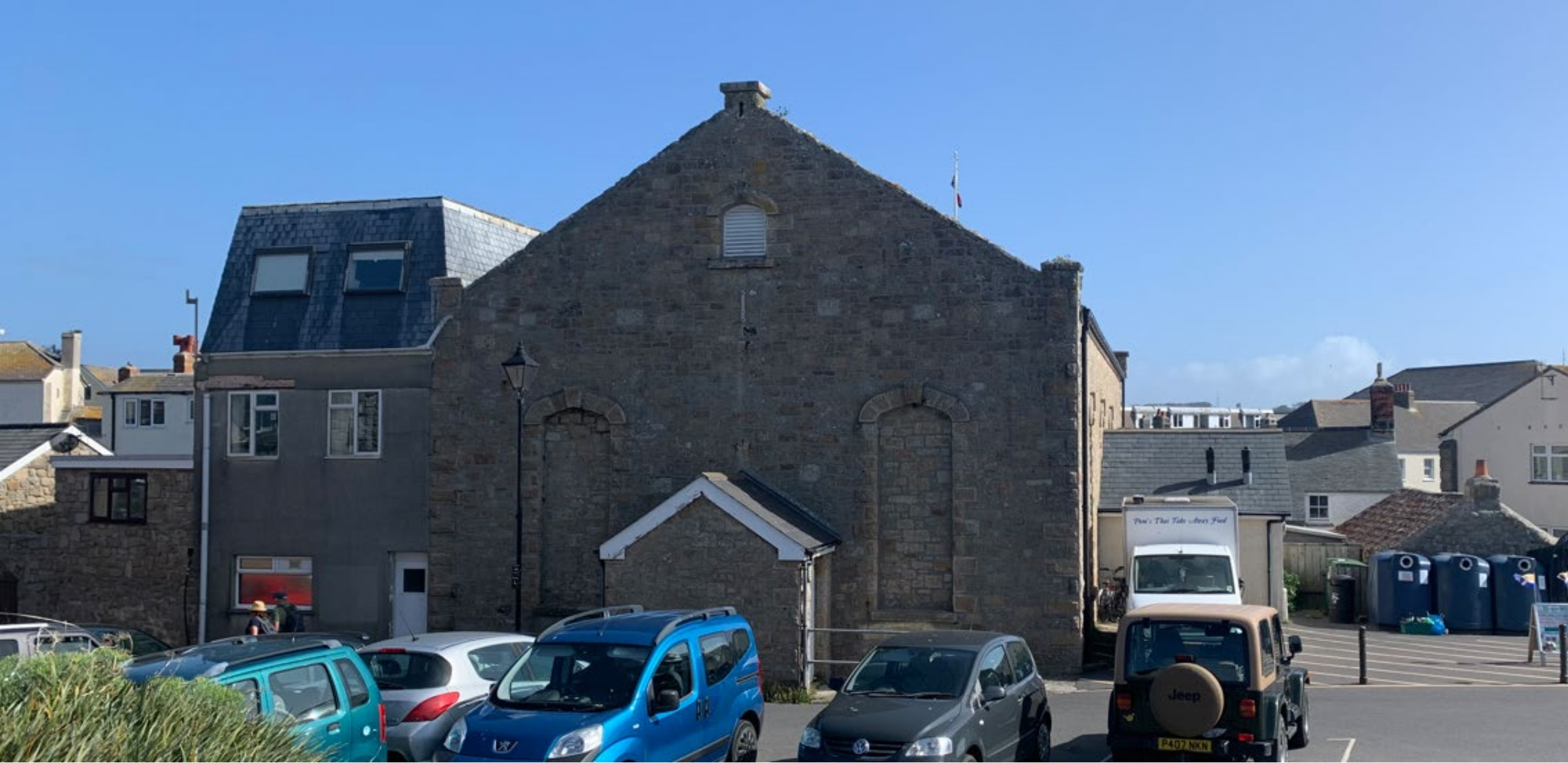
View of Existing Rear Elevation
