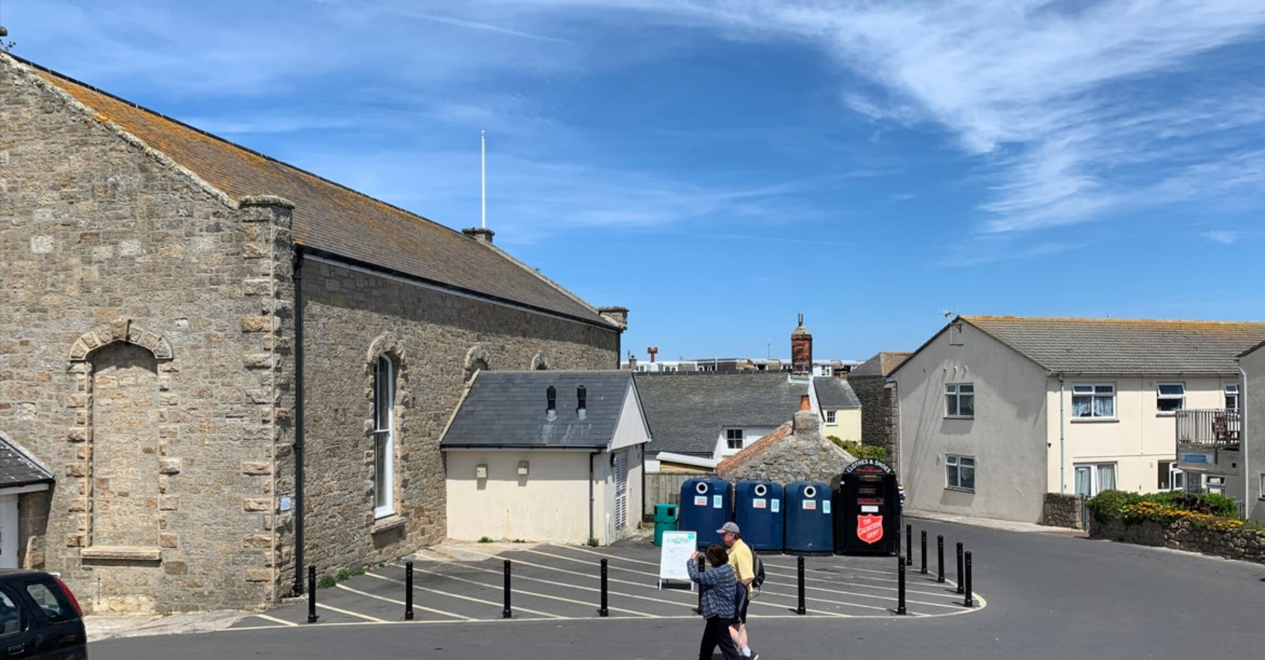
View towards the existing Side Elevation
