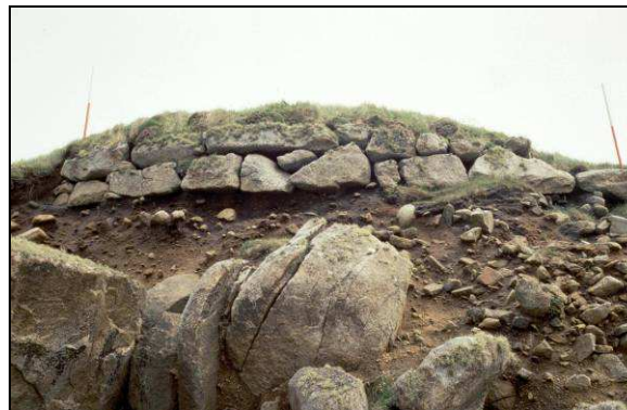
Fig 4.8 The front of a redan where the bank has been eroded to expose a wall face of two courses of large, trigged, angular boulders. Whether this is an original 17 th century wall or a later rebuild is not clear however the 2006 archaeological excavation suggests that it is an original feature. Given its parlous state the wall face is unlikely to survive many more severe storms. The friable nature of the cliff-face with the various densities of a stone/ boulder matrix is clearly visible with the granite bedrock protruding below (photo: EH)
