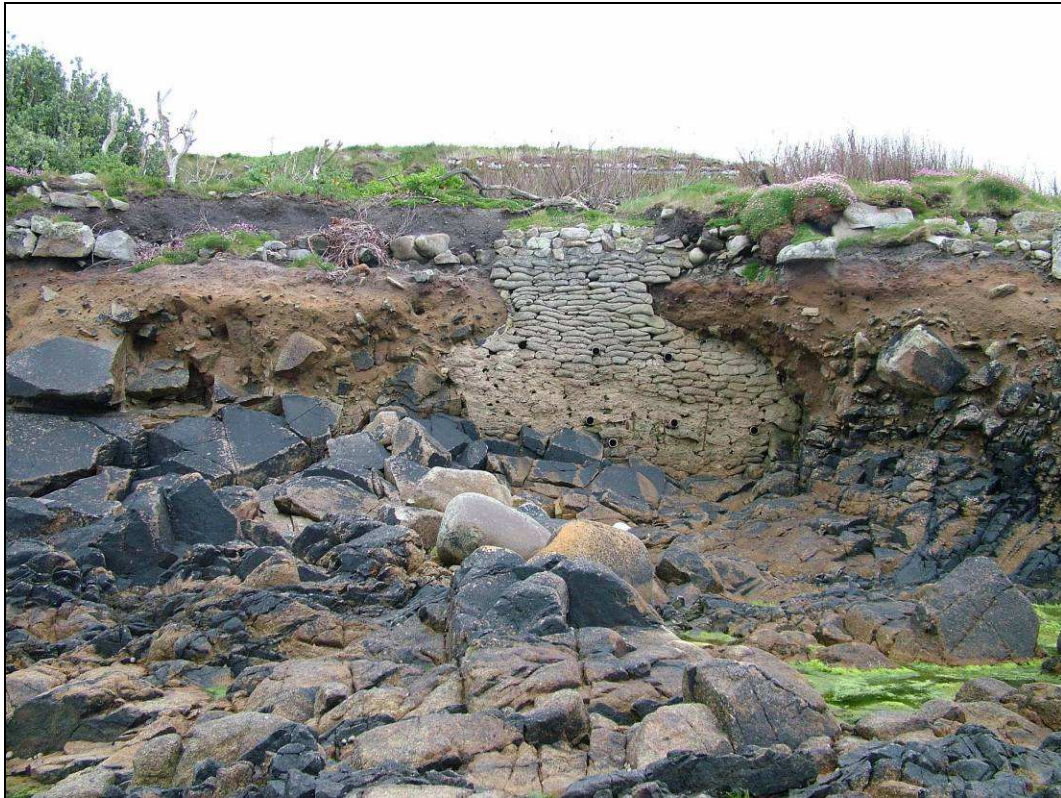
Fig 4.1 Repairs to a breach in the cliff face caused by wave erosion located to the east of King Charles' Battery (site 67). Note the scouring of the protective natural bedrock (and 'boulder field' that usually covered it) in front of the breach (photo: EH)
