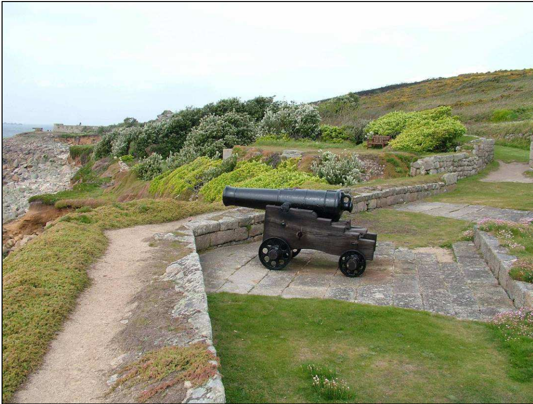
Fig 4.11 Erosion damage along the top of the wall at Morning Point Battery (the disused partly buried holding tank is visible beyond the top of the cannon)
