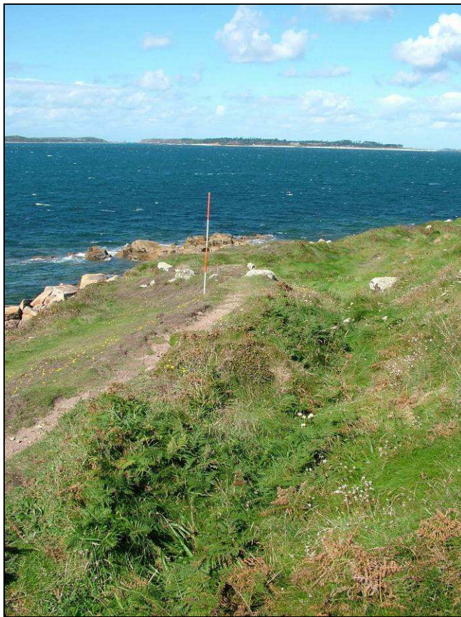
Fig 4.10 A footpath along the top of the 17 th century breastwork (photo: EH)
