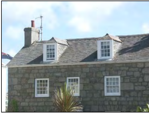
Coursed rubble stonework and slate-bung dormer cheeks: Riviera House, the Parade.
