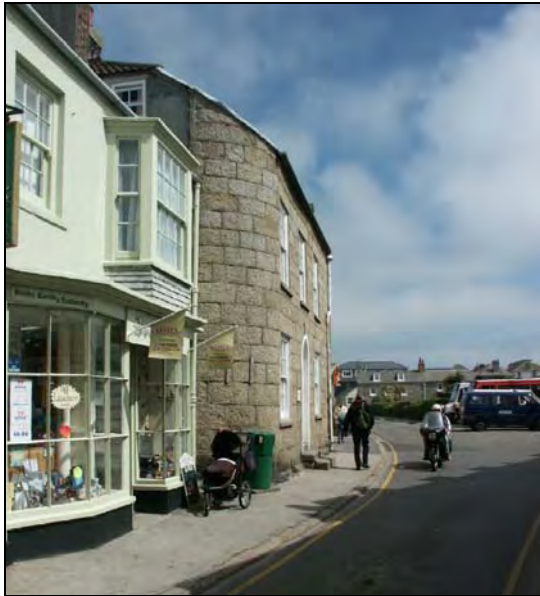
Fine stonework and a historic shop front at the west end of the Parade.
