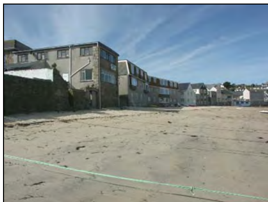
Town Beach – potential for reinstating character through an enhancement programme for elevations fronting the shore.
