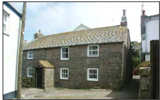
'Wahroonga', also known as Clemmies Cottage, Porthcressa Terrace. Coursed granite rubble and slate roof. Listed Grade II. An example of Hugh Town's surviving vernacular dwellings of the 18 th or early 19 th century.
