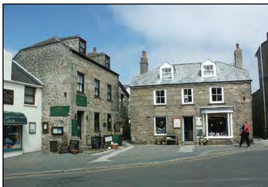
The 'square' at the east end of Hugh Street. Plain architectural forms, with good quality stonework to front elevations, rubble to the sides. The building on the right is one of a number of historic examples in Hugh Town of shopfronts inserted into domestic buildings.
