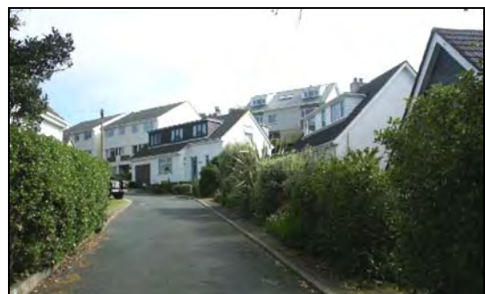
Dense 1960-70s development on a steeply sloping site at Rams Valley.
