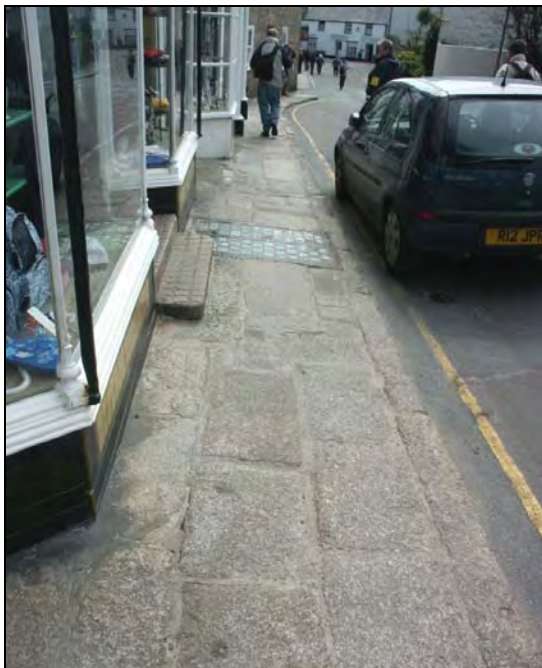
Distinctive surfacing. Left: Granite slab paving on the Bank. Right: a kerb of rough-dressed moorstone.
