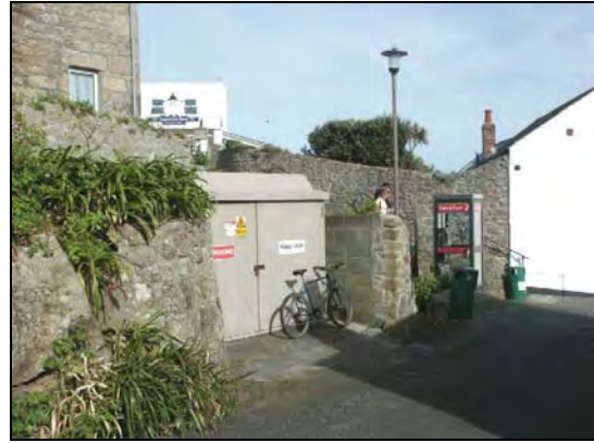
The foot of Garrison Hill – an opportunity to enhance the quality of the pedestrian approach to Hugh Town's major historic attraction.
