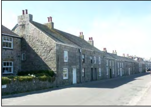
Plain 19 th century housing on Higher Strand, almost certainly associated with the shipbuilding industry located on the foreshore immediately in front.
