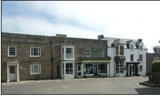
Elevations of coursed dressed granite and colourwashed render on the Bank.
