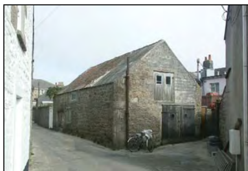
Historic outbuildings may offer potential for beneficial new uses.
