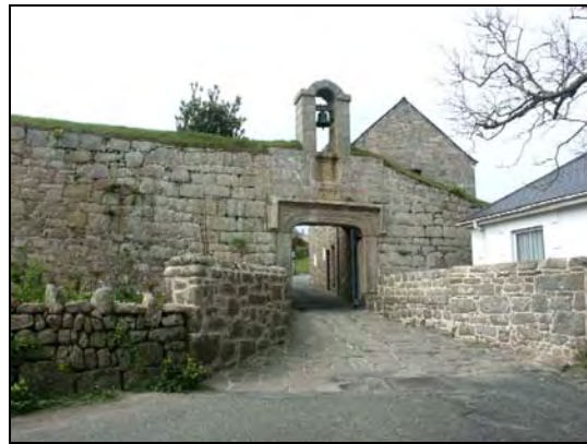
The Garrison gate. The bellcote was added to the late 16 th century gate to mark the expansion of the defences in the first half of the 18 th century.
