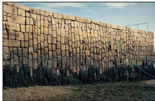
The distinctive stonework of the early 17 th century quay. (Photograph: Eric Berry.)
