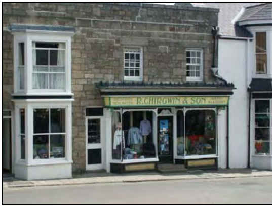
The English Heritage funded Isles of Scilly Grant Scheme aided refurbishment of this historic shopfront on the Bank.
