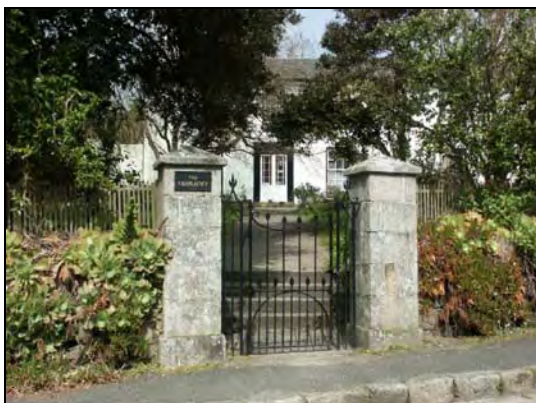
The gate to the Chaplaincy, Church Road. Greenery and good quality boundary features are characteristic of the area.
