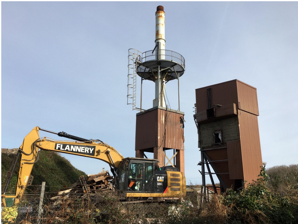
Figure 5 the 1970s incinerator during demolition in 2015
