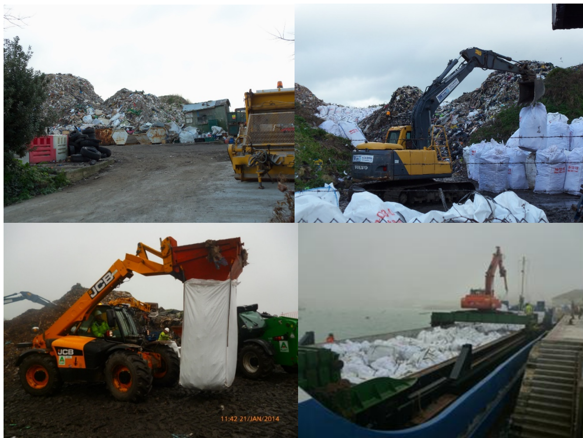
Figure 8 Images of the redevelopment of the waste site at Porthmellon 2015/2016
