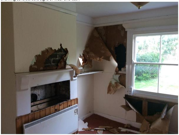
Built without a damp course, lacking insulation and constructed on a concrete plinth that is showing signs of salt intrusion the building as it is at present does not meet the standards required for rental either as a residential property or as premises for commerce.
