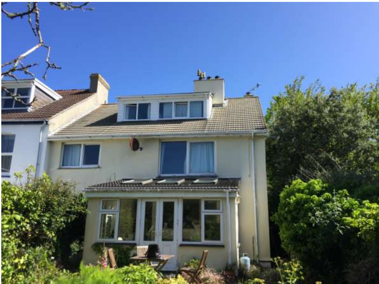
Figure 1 Rear Elevation of Property
