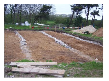
• An important high volume customer is St Mary's Riding Centre, then under construction. Here crushed aggregate can be seen in use constructing drains in the sand school
