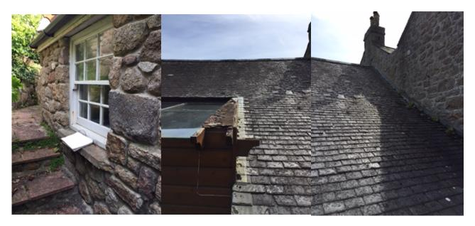
It would appear that roof profiles 1 & 2 have been renovated in the past as they both have bitumous or felt membranes below the tiles, this seems rather odd as the tiles themselves appear to be much older in parts. It is unclear whether roof profile 3 has ever been renovated as there is no membrane and the roof is scantle.
