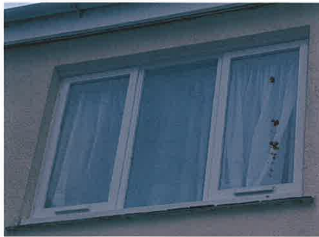
Existing rear first floor
