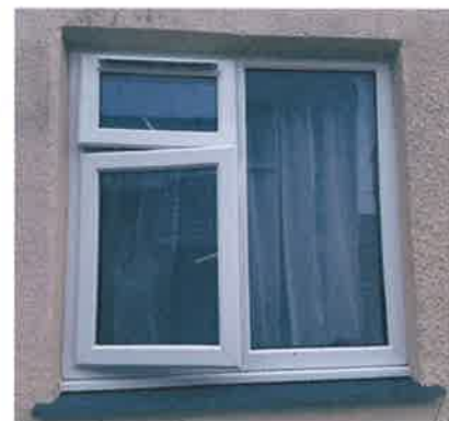
Existing rear ground floor
