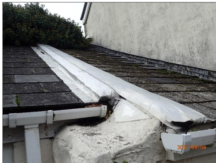
Single storey extension showing mis-aligned roof structures
