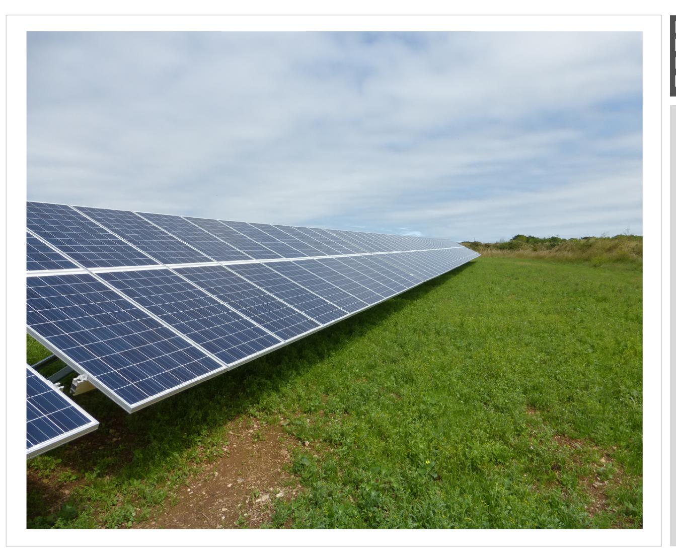
48.8kW Array, South orientation. Ten strings of 16 x 305Wp panels. Two 20kW 3phase dual MPPT inverters. Estimated annual generation of 49,000kWh
