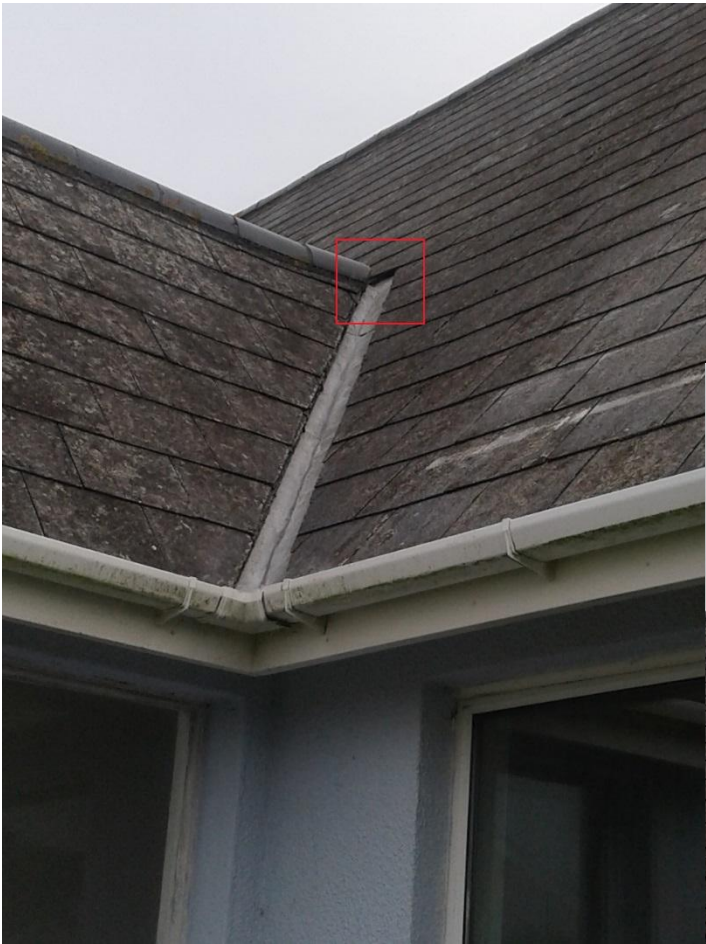
Photo 4b. Gaps under tiles overhanging valley and under final ridge tile.
