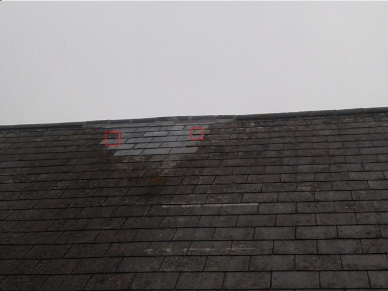
Photo 5. Raised roof tiles on main roof (western aspect)
