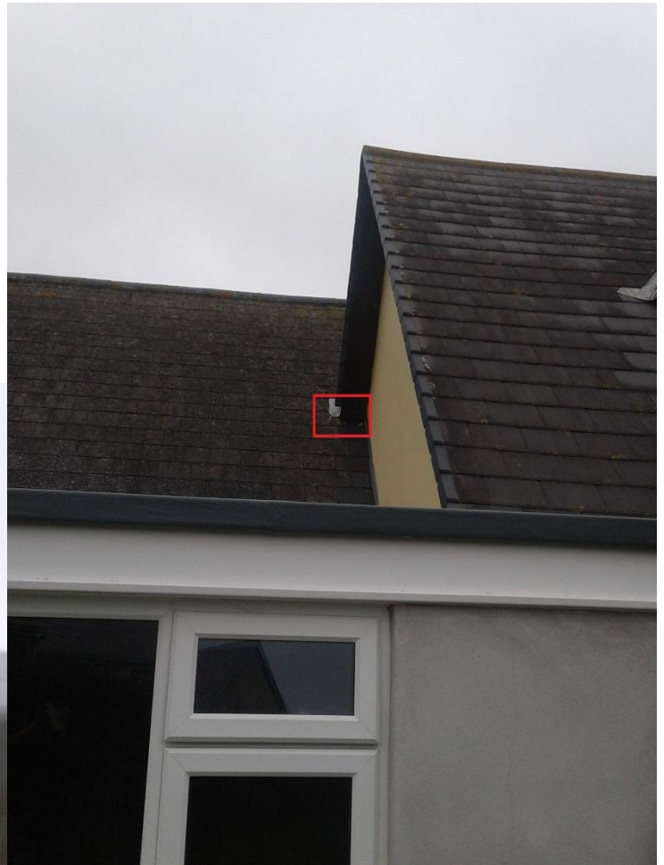
Photo 9. Gap in flashing
