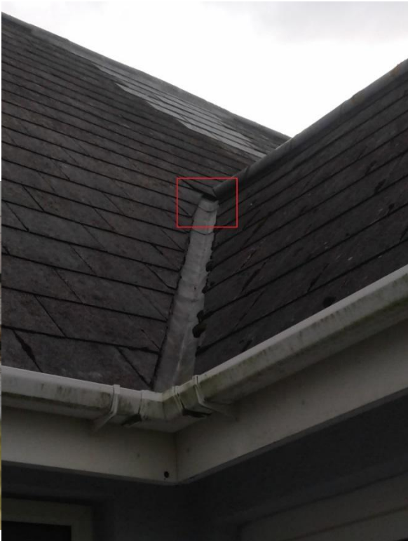
Photo 4a. Gaps under tiles overhanging valley.
