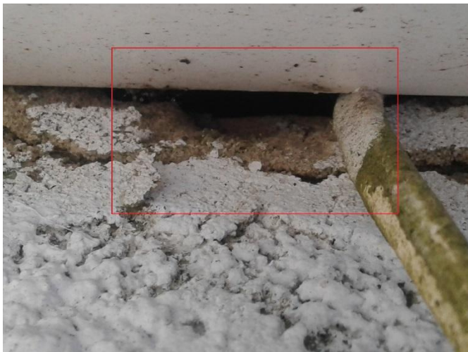
Photo 3. Gap behind the soffit where the cable runs,
