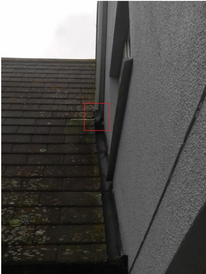
Photo 1. Gap in flashing and under soffit
