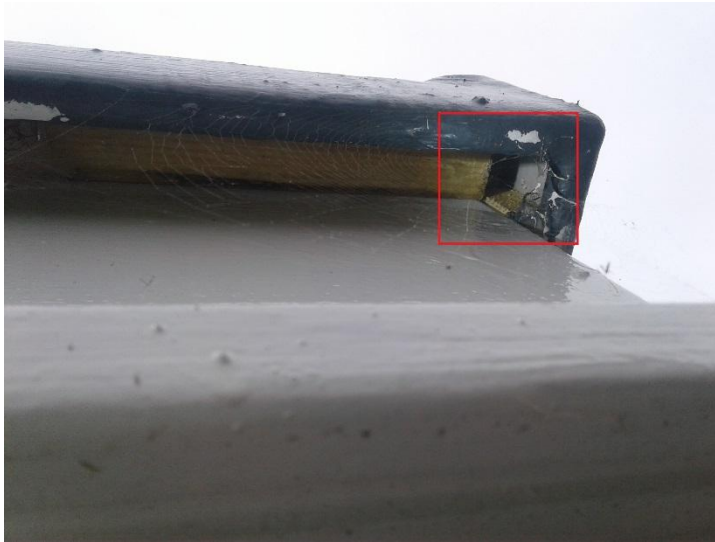
Photo 8. Gap between battens
