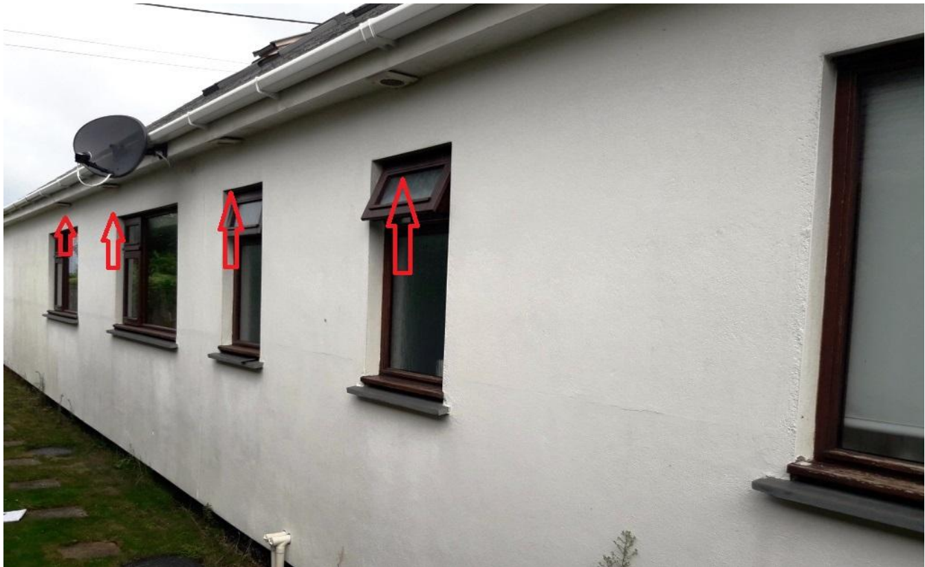
Photo 5a. Location of vents in southern aspect soffit board
