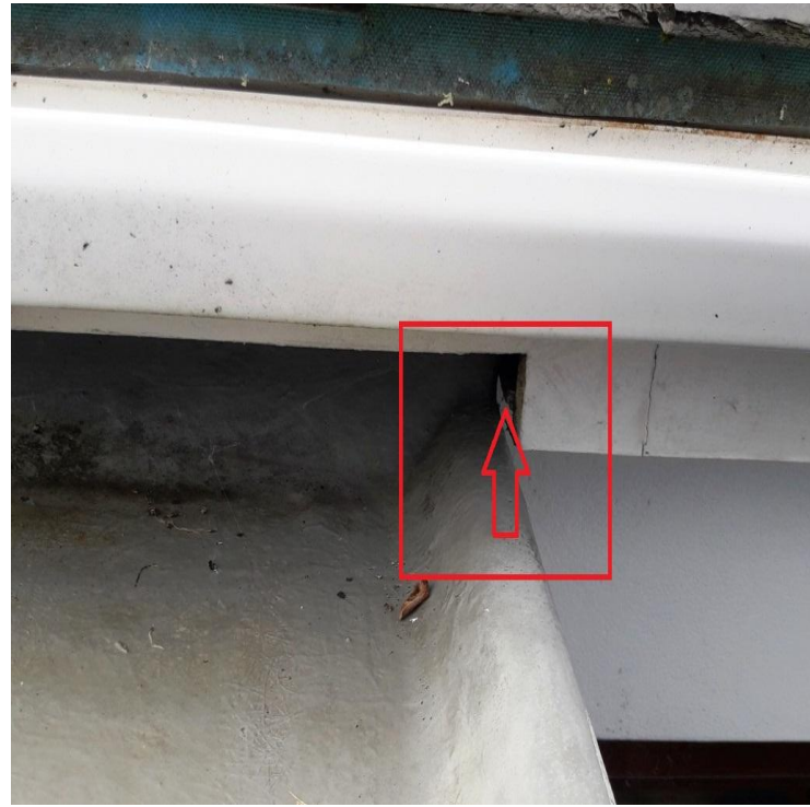
Photo 6a. Gap behind fascia taken from above garage roof
