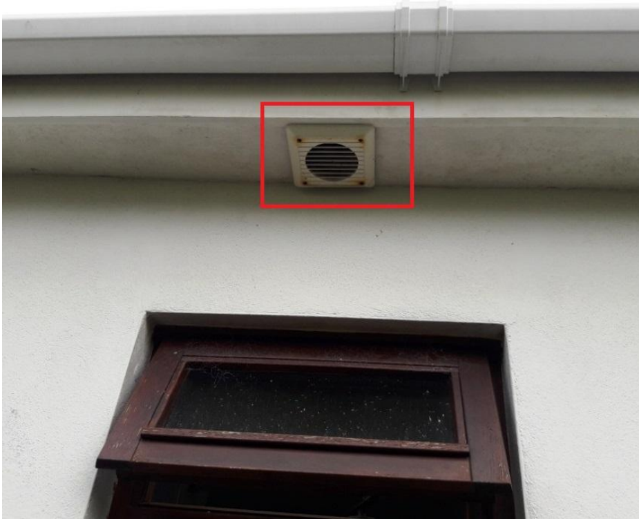
Photo 5. Close-up of vent in southern aspect soffit board
