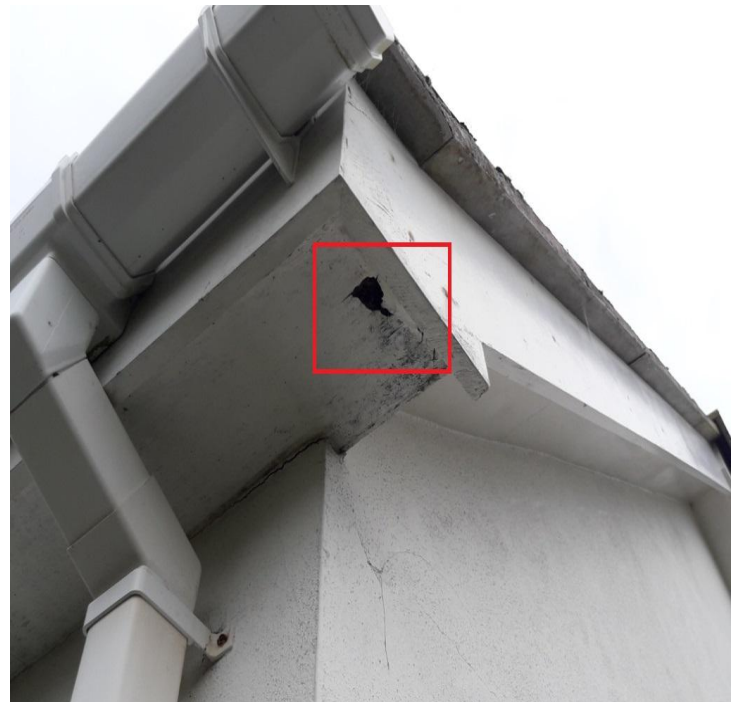
Photo 4. Small hole in soffit in south aspect of single storey extension
