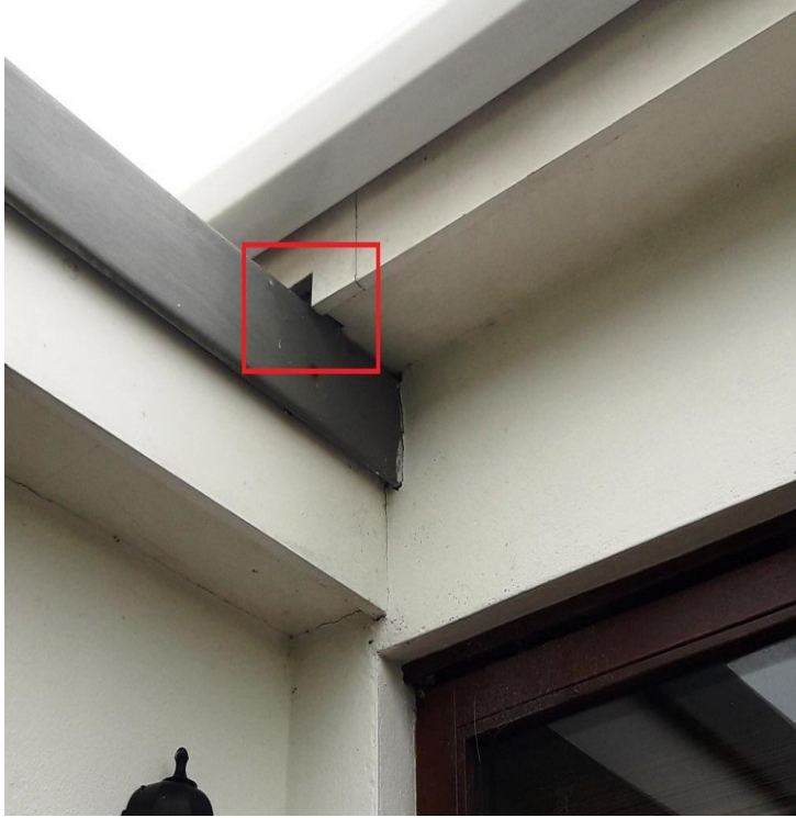
Photo 6. Gap in fascia and soffit where garage joins the northern aspect of the main dwelling
