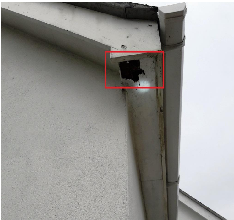
Photo 3. Piece of soffit missing in north aspect of single-storey extension
