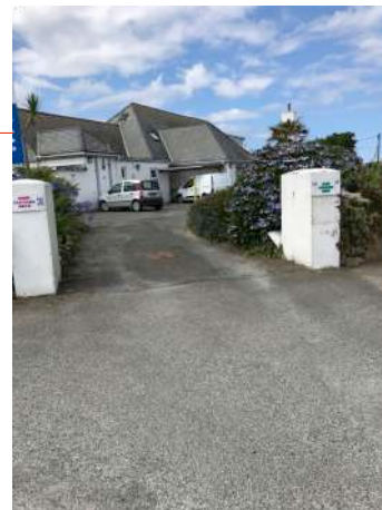
Photograph 1 Indicating main entrance view from public highway
