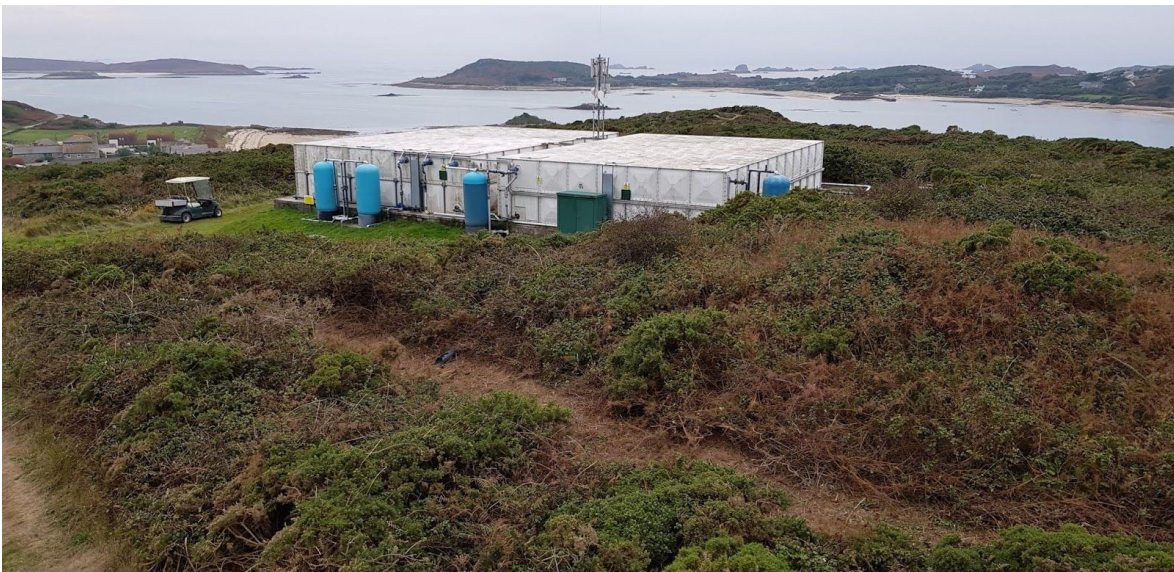
Plate 6: The reservoir on the summit of vane hill. Cairn 'B' is visible as the slight mound on the right of the image and the boundary of the SAM (3) within which it sits extends to roughly half-way along the right-hand water tank. Cairns 'C' and 'D' (1 & 2) are on the far side of the reservoir.
