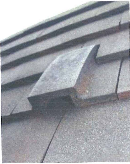
Figures 3. Example of an in-line roof tile (tailored to your roof material style and its placement within the roof)
