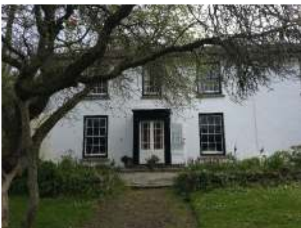
Photograph 3 – Porch front elevation
