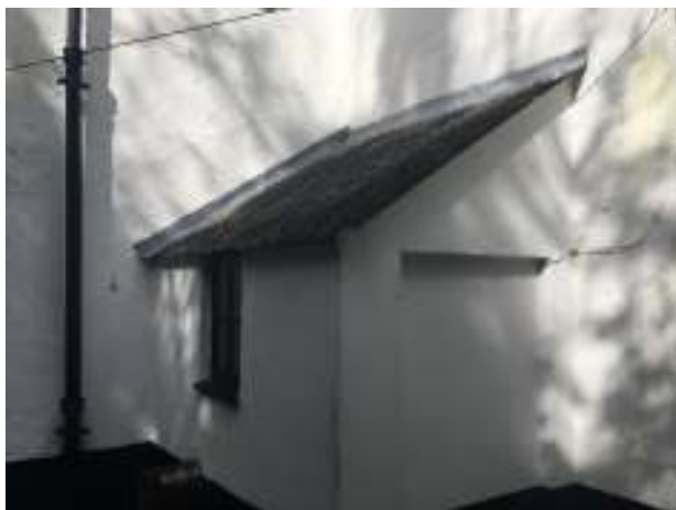
Photograph 1 – Plant room External
