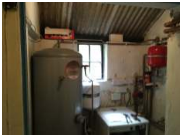
Photograph 2 – Plant room Internal
