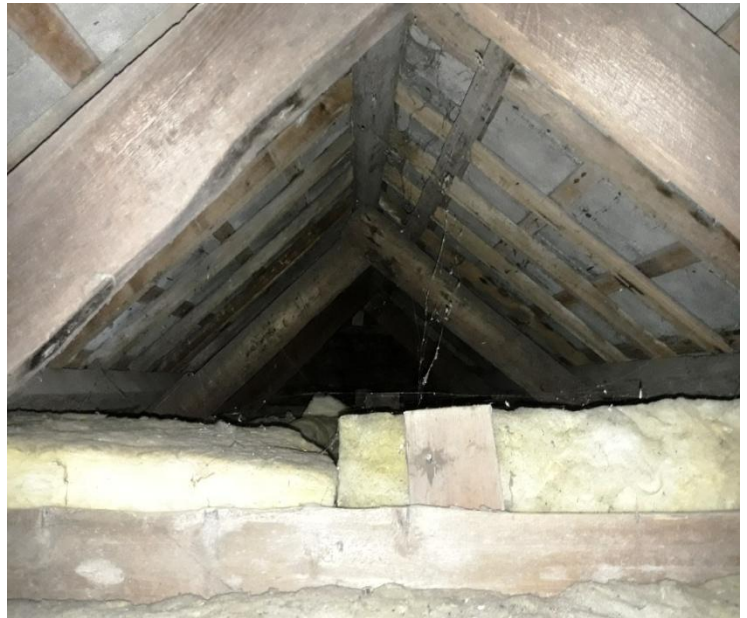
Photo 14. Two-storey loft space
