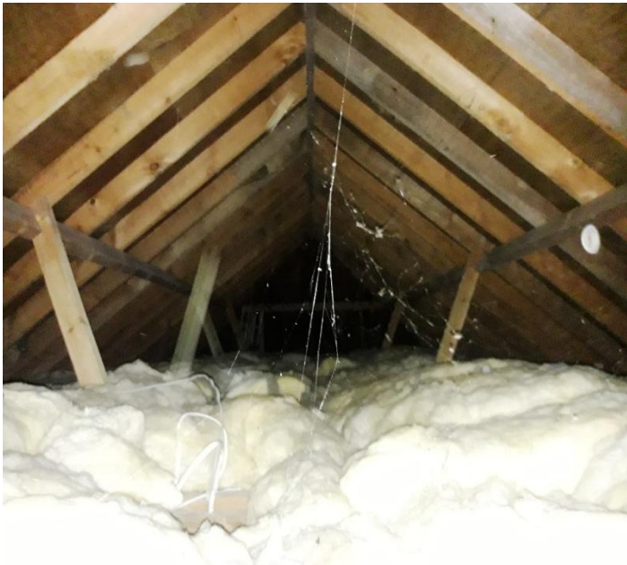
Photo 13. Single-storey loft space
