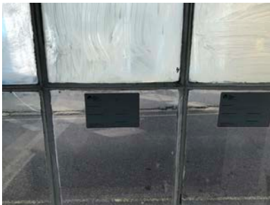
Window Moulding (Inside View) Showing internal Putty to Glazing
