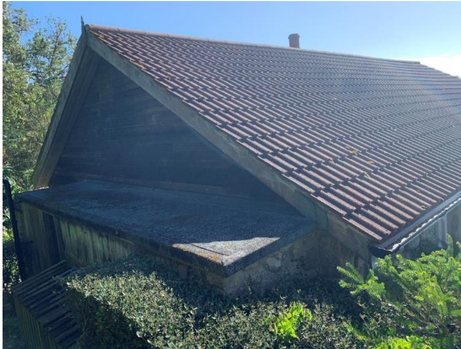
Figure 4: View of the north elevation of the Racket Town.
