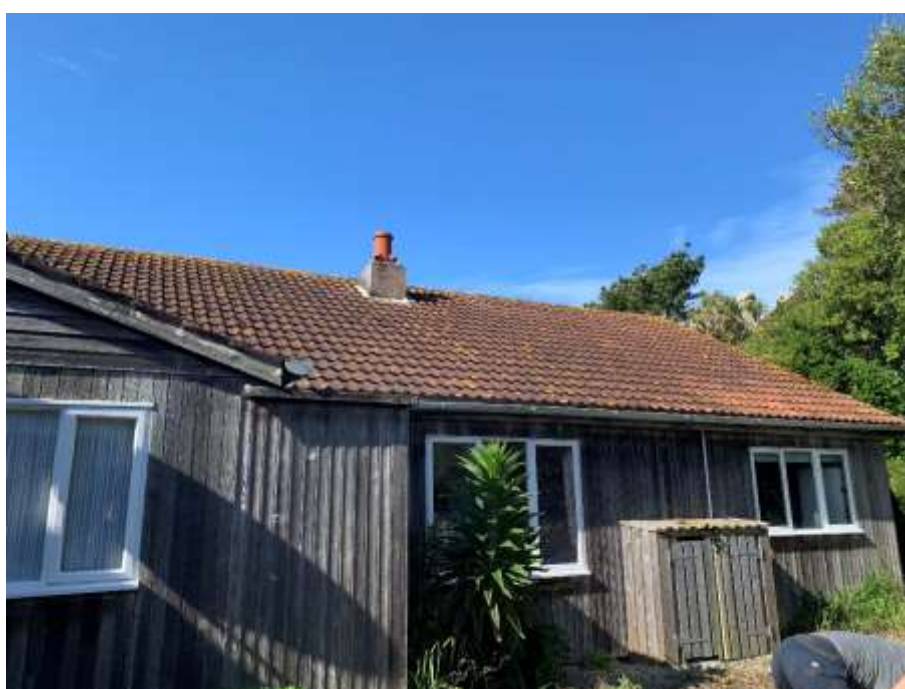
Figure 2: View of the east elevation of Racket Town.
