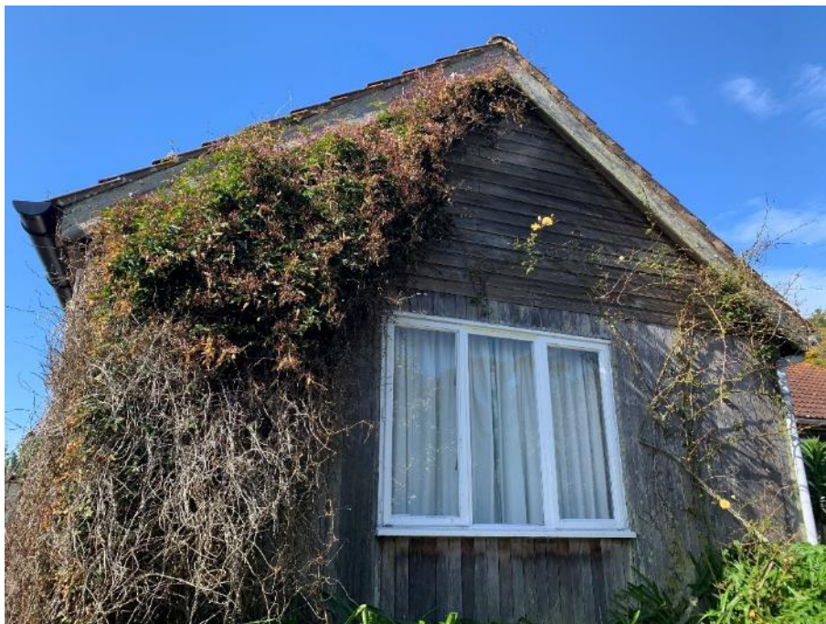
Figure 5: View of the eastern elevation of the south-east projection of Racket Town, showing dense ivy.
