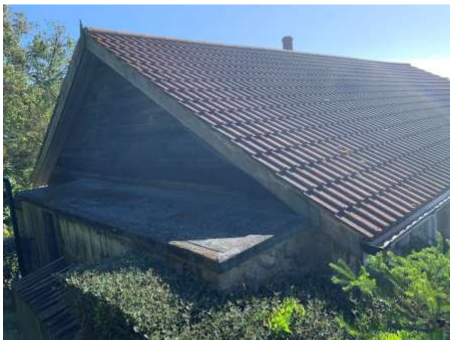
Figure 3: View of the north elevation of the Racket Town.
