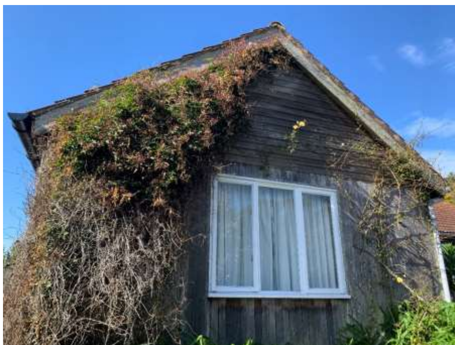
Figure 4: View of the eastern elevation of the projection of Racket Town, showing dense ivy.
