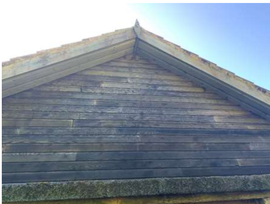
Figure 6: View of the cladding and the wooden facias and soffits on the north elevation of Racket Town.
