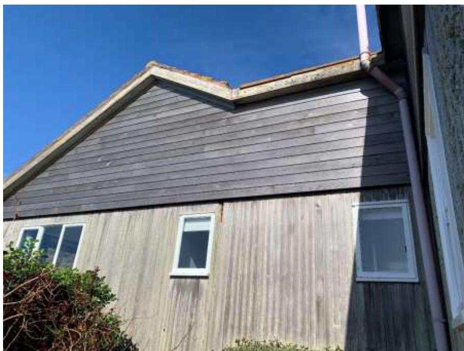
Figure 5: View of the north elevation of the projection of Racket Town.
