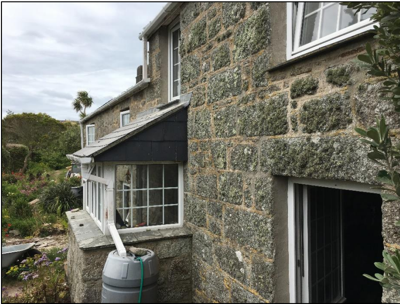
Photo 01 – showing the well-pointed granite exterior and well-sealed uPVC window characteristic of the building.
