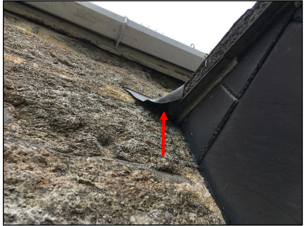
Photo 05 – showing the lifted flashing where the roof of the porch meets the wall – the gaps beneath the fascia/barge boards illustrated in Photo 02 are visible above.
