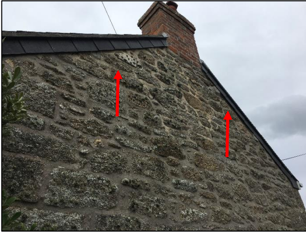
Photo 04 – showing the eastern gable of the building with hanging tiles along the verge and a well-pointed granite external wall. The brick-built chimney is also visible.
