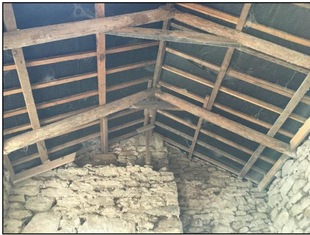
Photo 06 – showing the interior of the building, open to the rafters and built around a wooden A-frame structure
