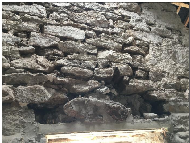
Photo 09 – showing gaps in the stonework internally.
