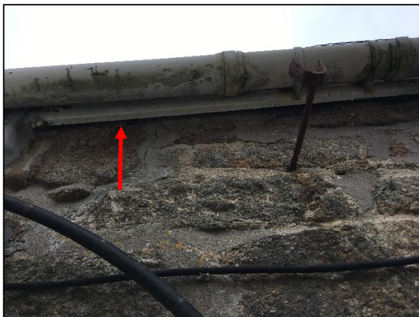
Photo 02 – showing the lifted fascia/barge board providing potential access behind – this is an example of a feature which is ubiquitous along eaves of the building.
