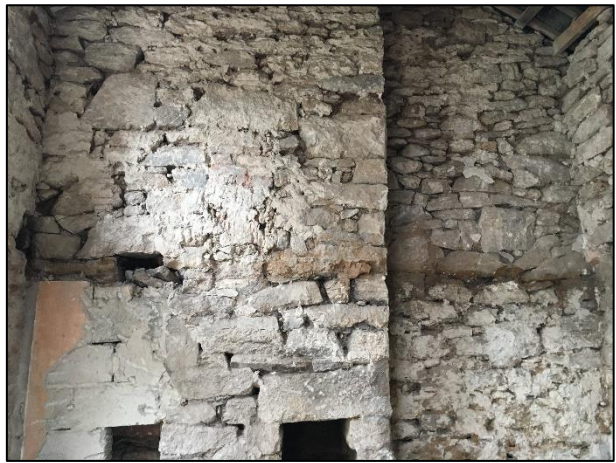
Photo 07 – showing the unfinished interior walls with multiple gaps between stonework.
