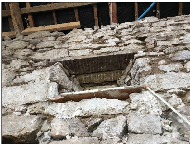
Photo 08 – showing gaps associated with lintels around a window frame
