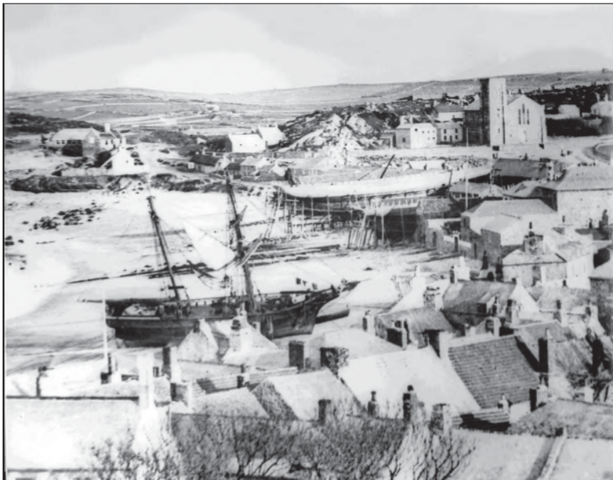
Fig 2 Shipbuilding on Town Beach, c 1870 (© Gibson Collection).
