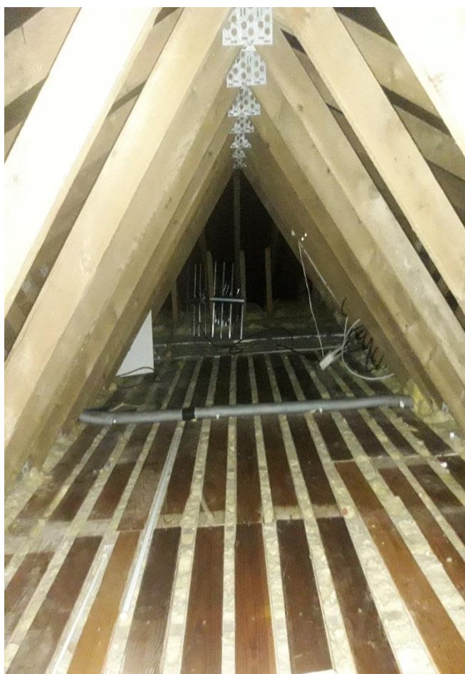
Photo 3. View of internal roof space and modern roof truss construction
