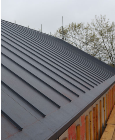
Single ply membrane roof
