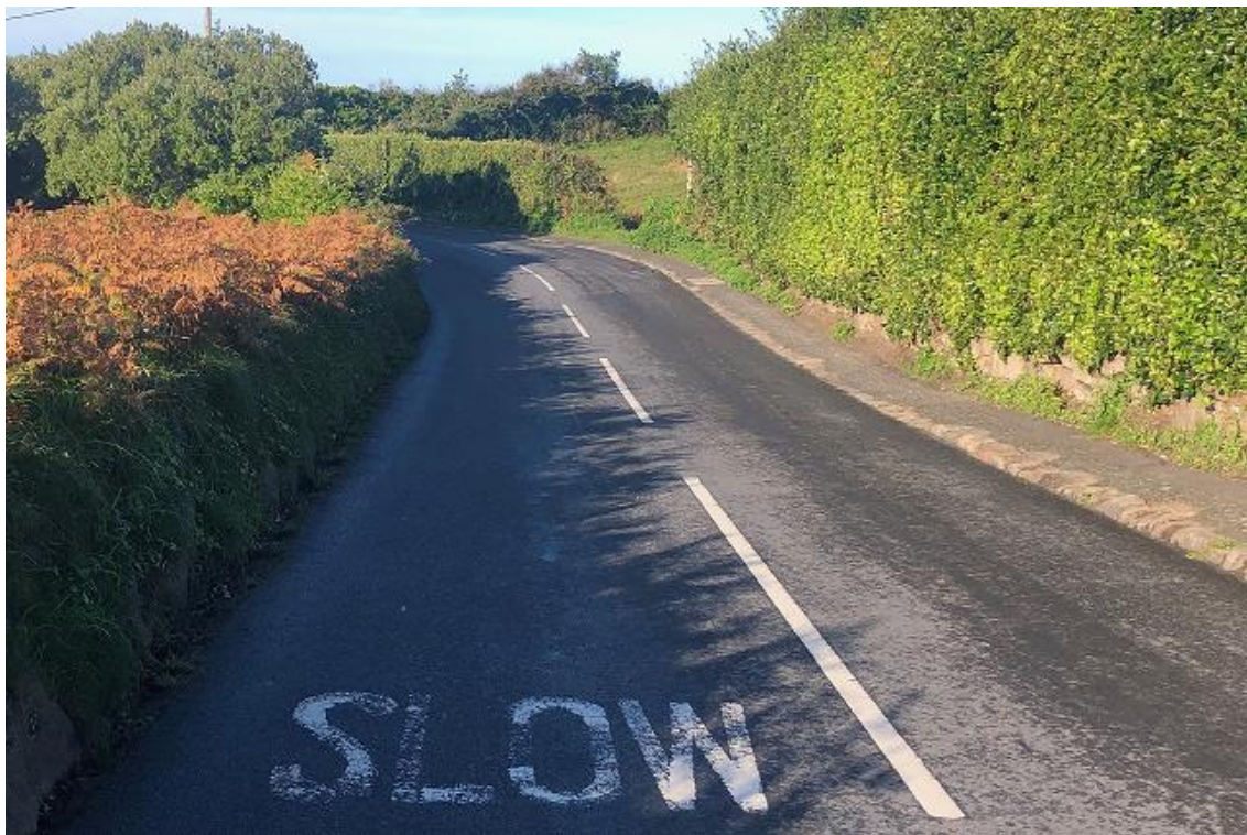
Plate 2 – Westbound Approach to Speed Reducing Corner With 'Slow' Marking
