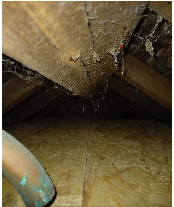
Photo 7. Internal loft space behind Velux window
