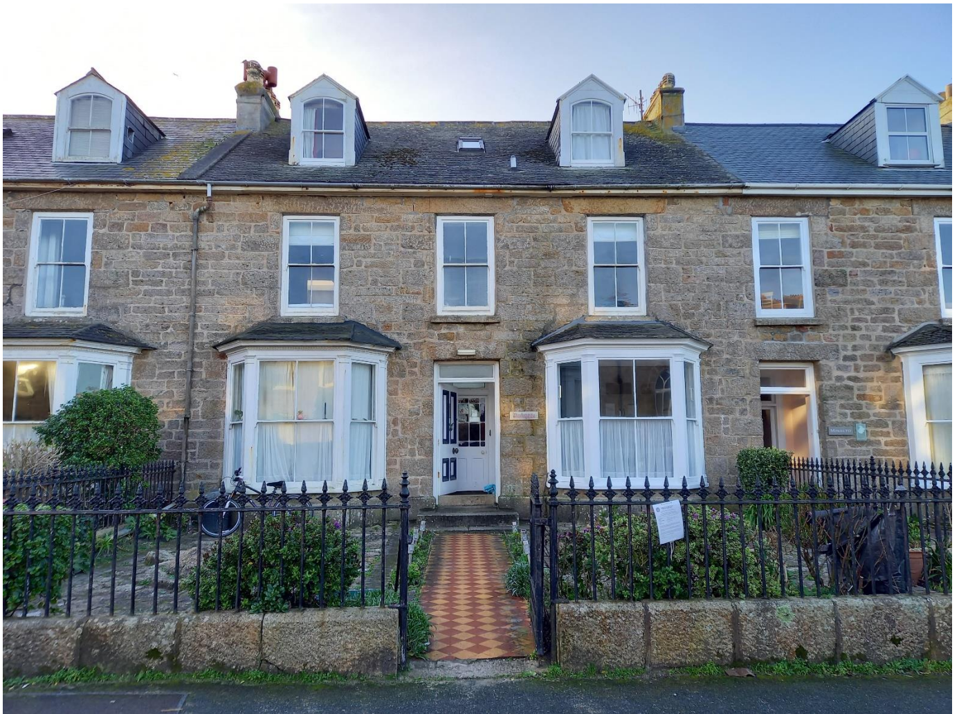
Photo 1. North Elevation of Warleggan Flats
