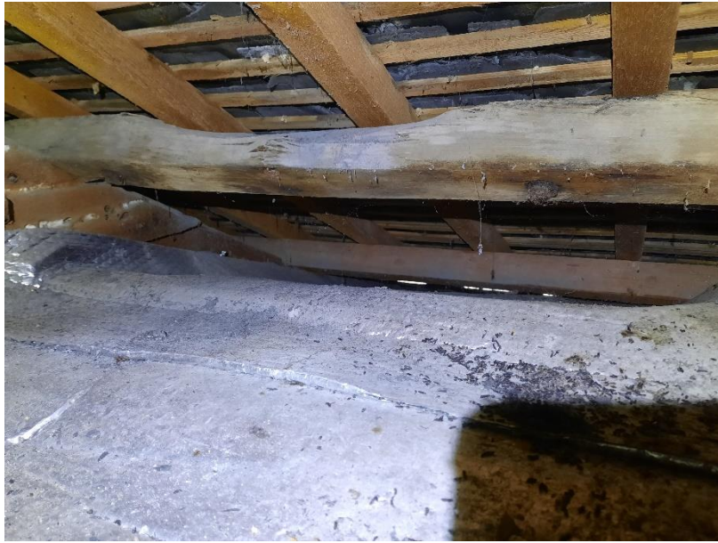
Figure 11: View of gaps at the wall tops of void 4 within cottage 3
