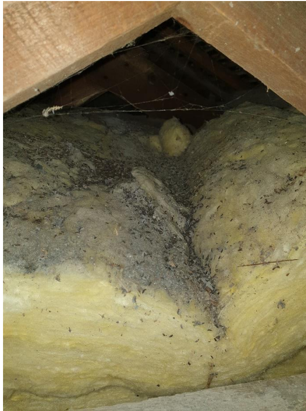
Figure 9: Accumulation of bat droppings within void 3, cottage 2 (viewed towards the east).
