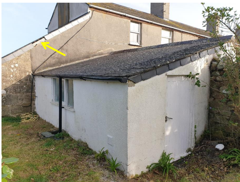
Figure 7: Southern and western elevation of outbuilding 1, also showing hole in roof from missing hanging slate on cottage 1 lean-to (yellow arrow)
