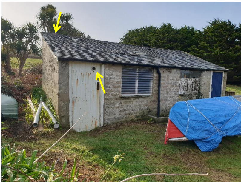
Figure 13: Northern elevation of detached outbuilding, showing holes in door and roof (yellow arrows)
