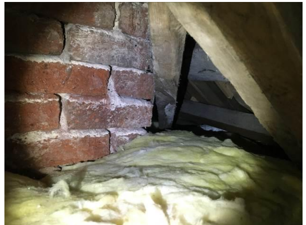
Photograph 4: Showing the chimney from within the roof space of Freesia guesthouse – the brickwork is well pointed and no cavities were noted.
