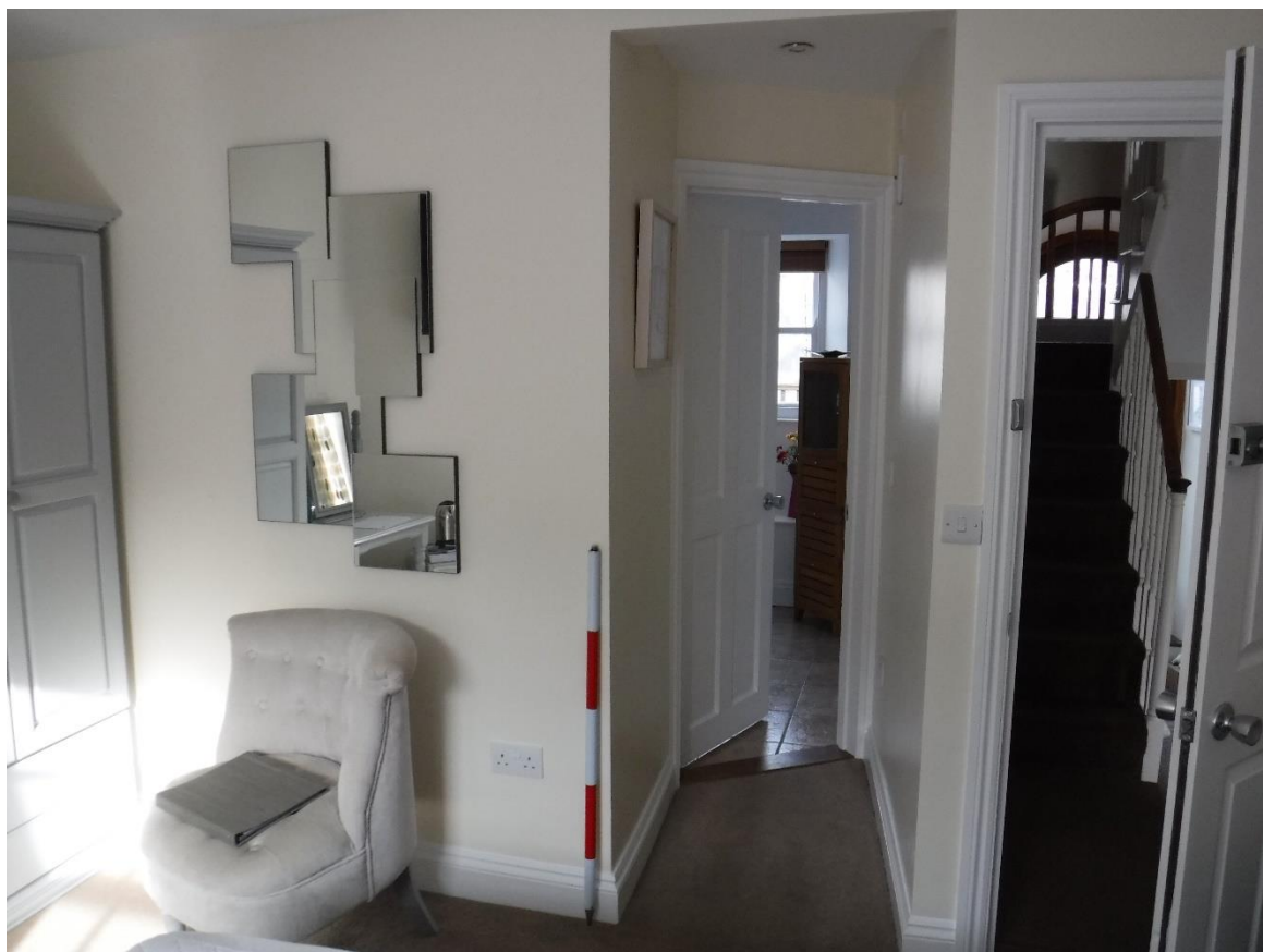
Fig 15 Stud wall concealing chimney breast on first floor.
