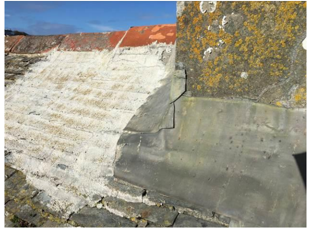
Photograph 2: An example of the tightly fitted flashing where the concrete-rendered chimney meets to the roof of Bordeaux.
