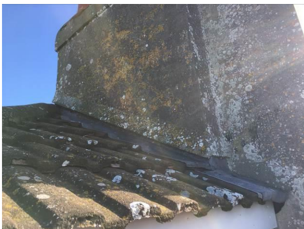
Photograph 5: Showing the well-fitted concrete roof tiles of Freesia abutting the chimney.
