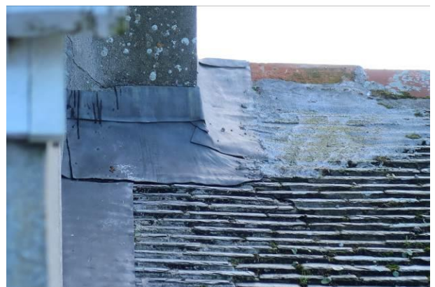
Photograph 6: Showing the well-fitted scantle slate tiled roof of Bordeaux.
