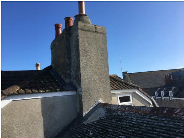
Photograph 3: Showing the hipped roof on the gable end of Freesia with the chimney meeting the lower roof of Bordeaux.
