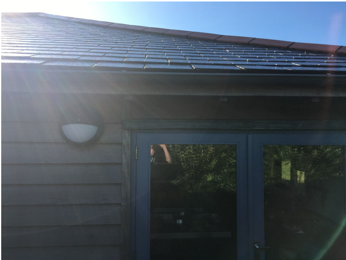
Rear doors of Island Fish where the Work Room will be attached
