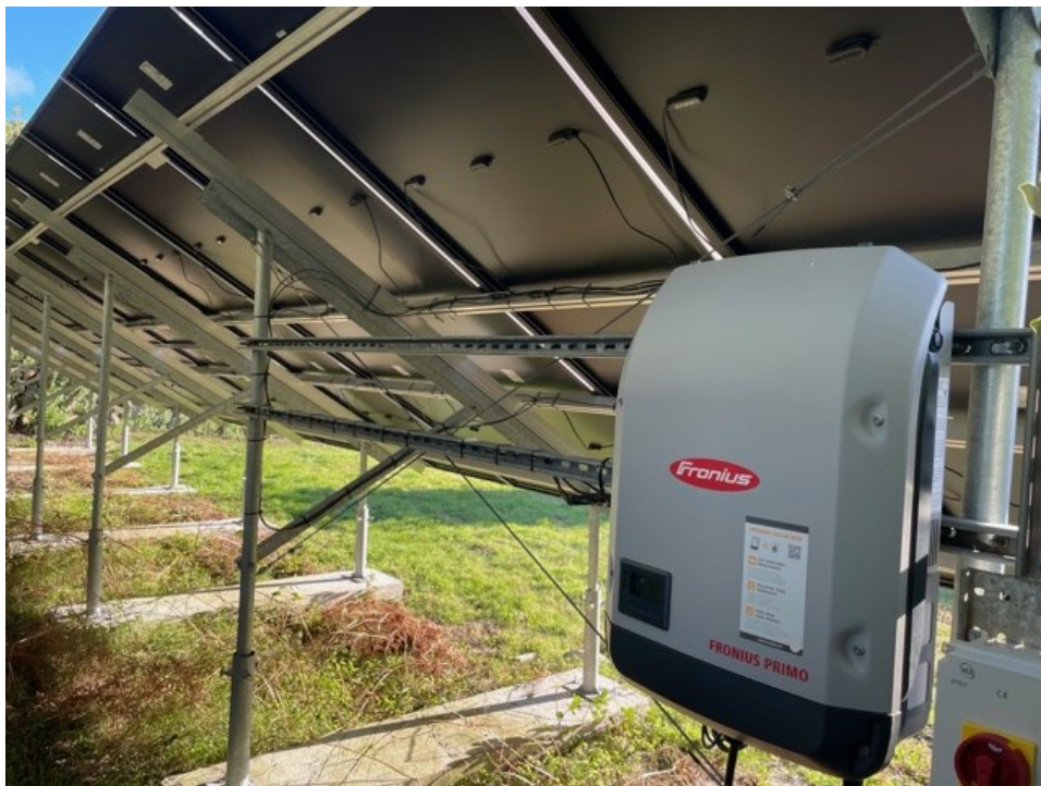
Figure: Showing the small concrete pads which would comprise the ground-works required to support the PV array with the inverter and battery situated beneath
