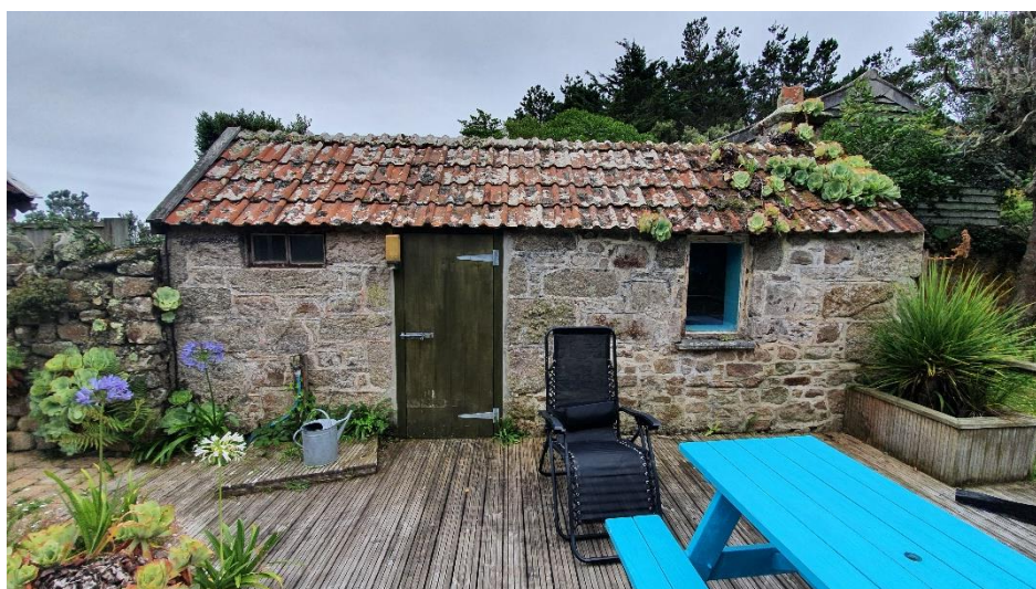
Figure 6: Northern elevation of detached outbuilding
