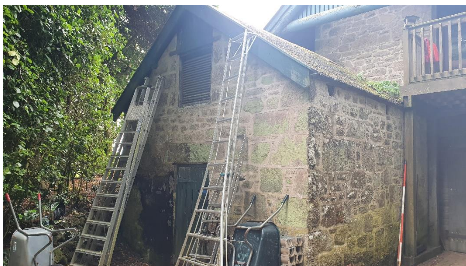
Figure 5: Northern elevation of attached outbuilding
