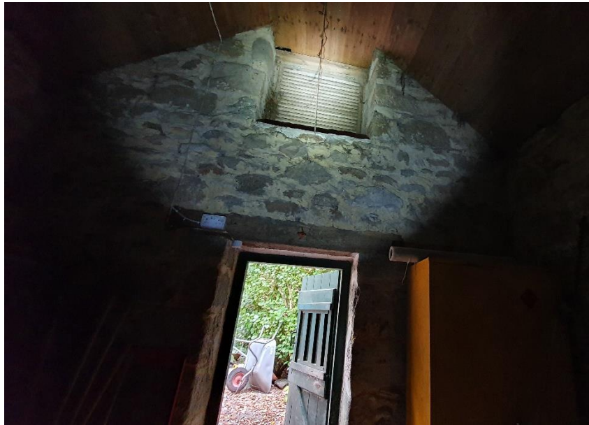
Figure 13: Interior of attached outbuilding (viewed towards the north).
