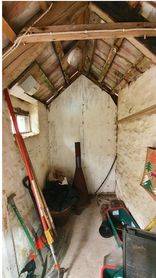
Figure 14: Interior of eastern room within detached outbuilding (viewed towards the east).
