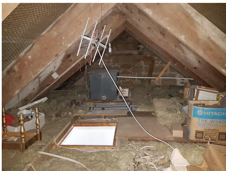
Figure 10: Interior of roof void over apartment (viewed towards the south)
