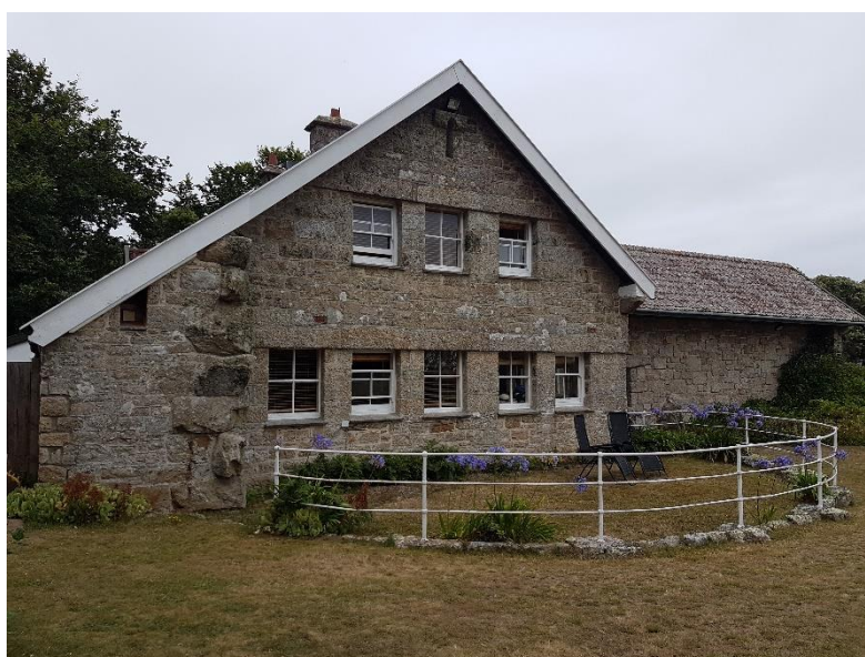
Figure 2: Southern elevation of Valhalla
