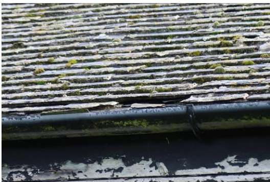
Photo 09 – Showing an example of the minor gaps in the tiles; otherwise the scandle tiles are well fitted with mortar beneath.
