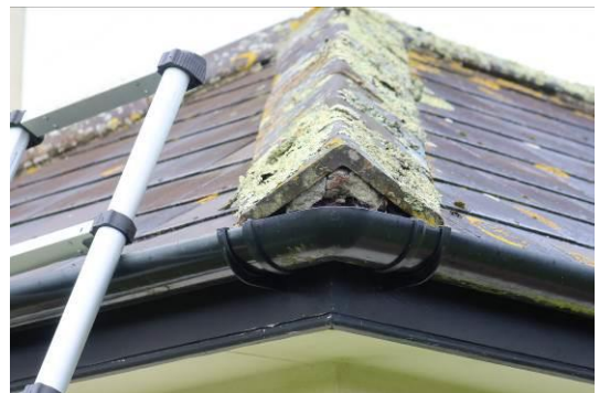
Photo 10 – Showing the damaged terminal hip tile in the south-east corner of the property – this was inspected at height and no roosting potential was identified.
