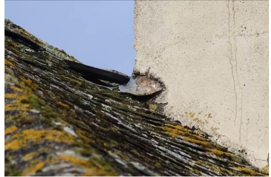
Photo 08 – Showing the slightly lifted flashing around the chimney – this appears to be superficial
