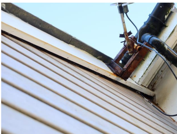
Photograph 5: Showing the fascia board on the north-western gable with gaps beneath. This area would not be directly impacted by proposals.
