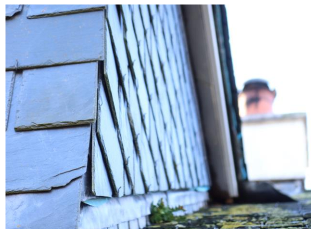
Photograph 6: Showing the slightly lifted tiles on the adjacent dormer with the lifted flashing where it meets the main roof visible to the right.
