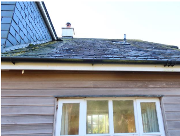
Photograph 3: Showing the roof section taken from the rear of the property – the tightly-fitted wood cladding of the exterior can be seen.
