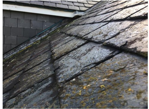
Photograph 2: Showing the roof structure from the existing Velux window – the scallie tiles are well fitted and in good condition. The adjacent dormer can be seen in the background.
