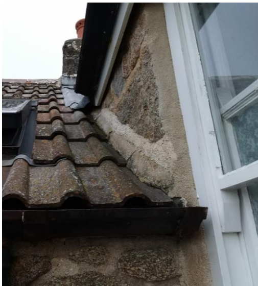
Photo 7. Showing the point where the house and barn join and an example of the gaps behind the fascia board
