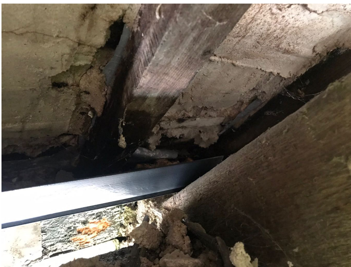
Photographs courtesy of the Duchy of Cornwall showing the temporary repair above the bathroom window to provide drainage
