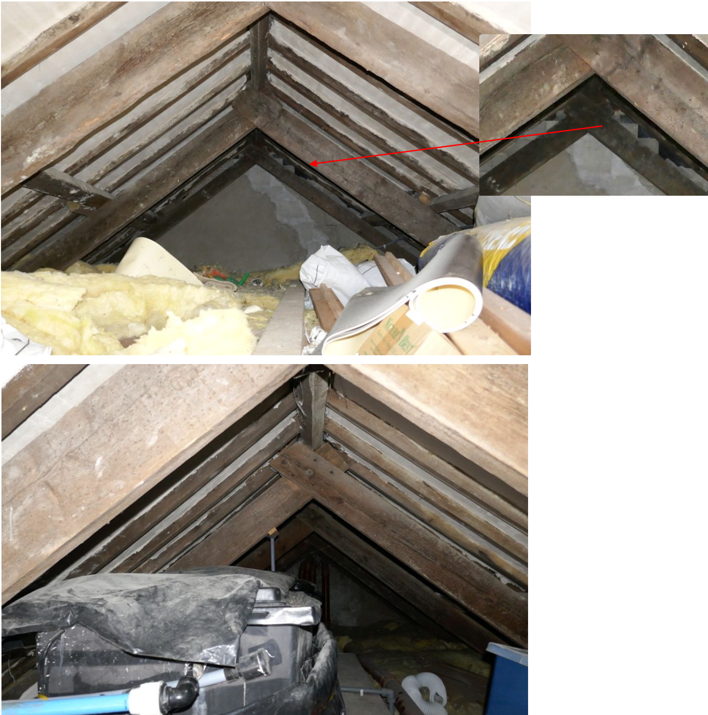
Top: Roofspace looking to the rebuilt south elevation showing incomplete infill to the west side
