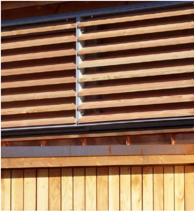
Fixed timber louvres to allow for ventilation and to control direct sunlight
