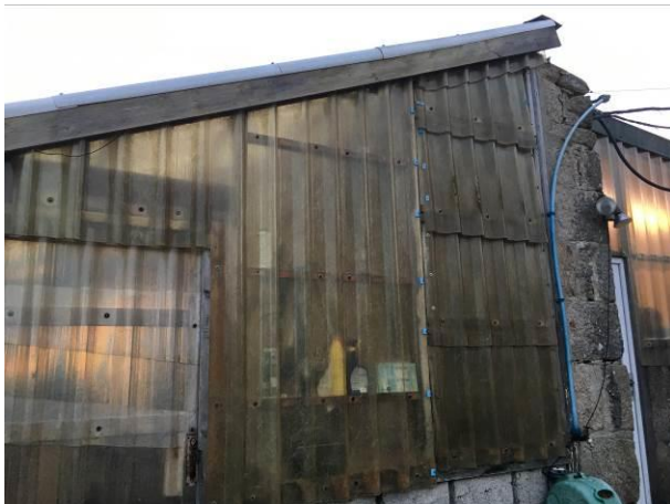
Photograph 5: Showing the eastern gable of the existing glasshouse with the translucent corrugated panels forming the majority of the structure.
