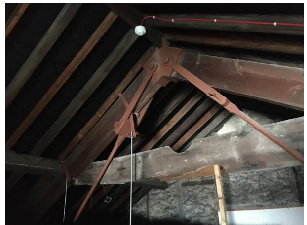
Photograph 12: The attic space within the main hall showing the timber roof structure and underfelting above. Lighting is from the window set into the north wall.
