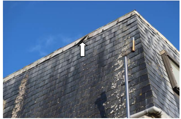
Photograph 8: Showing an example of lifted flashing at the top of the hanging tiles on the 1970's extension.
