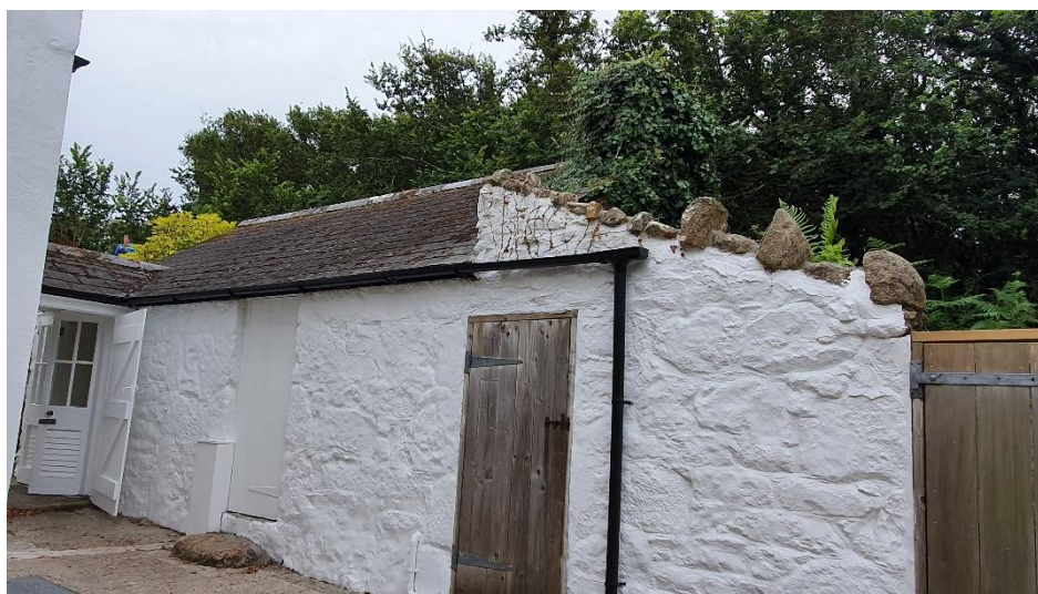
Figure 4: North-eastern elevation of outbuilding and part of roofless structure
