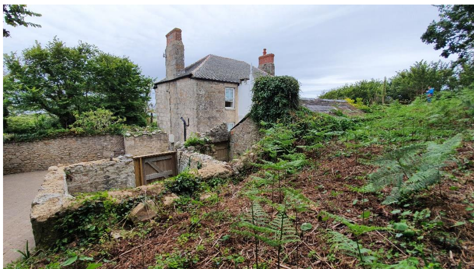
Figure 5: South western elevation of Dolphin House and roofless structure (viewed from top of earth bank)
