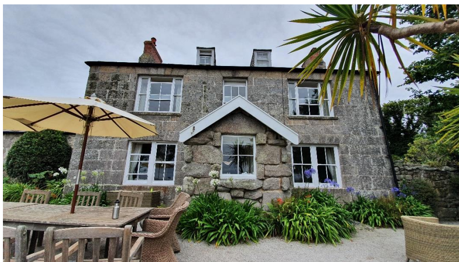
Figure 2: North-eastern elevation of Dolphin House
