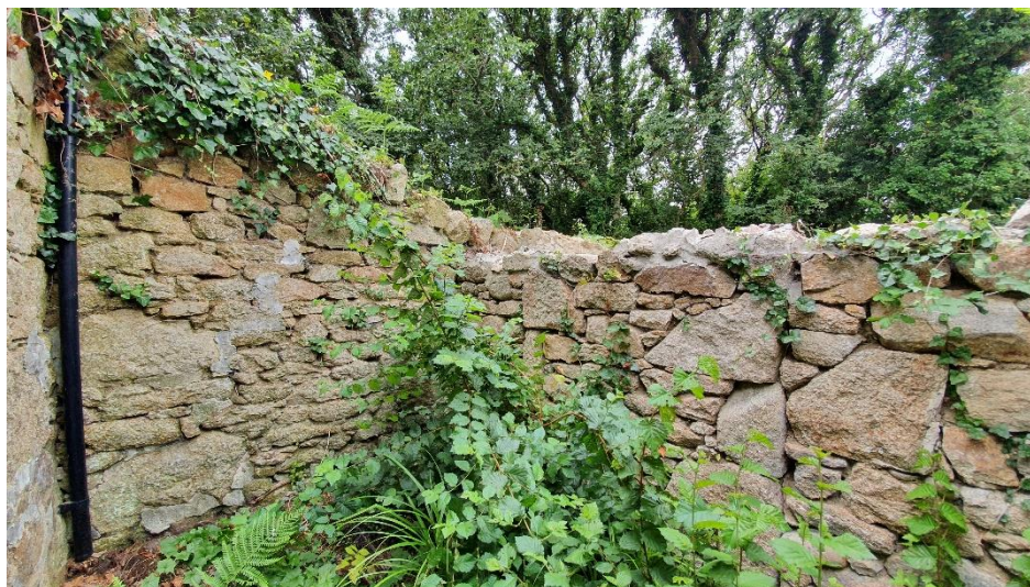
Figure 8: Interior of roofless structure (viewed towards the north-west)
