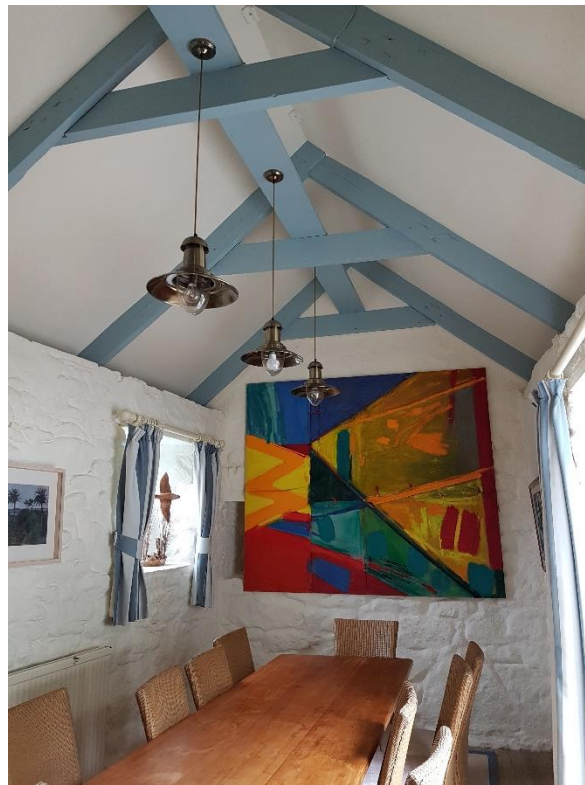
Figure 7: Interior of single-storey extension (viewed towards the south-east)
