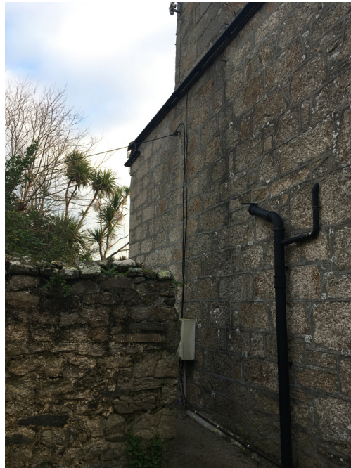
Figure 7 - North west elevation of Dolphin House (LHL)
