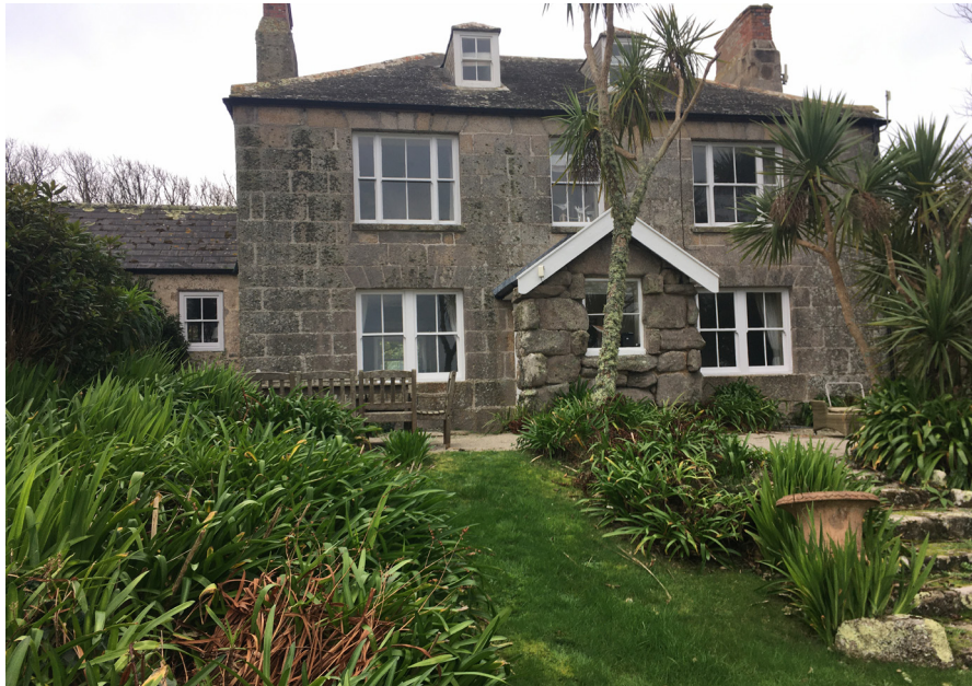
Figure 5 - Front elevation of Dolphin House (LHL)
