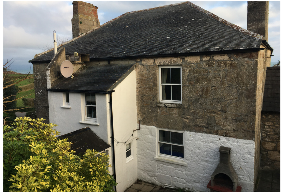
Figure 6 - Rear elevation of Dolphin House (LHL)
