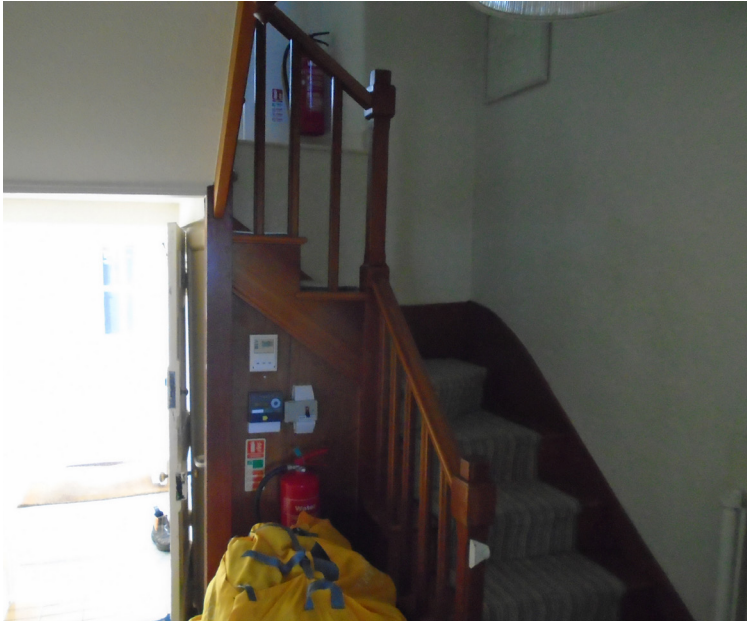
Figure 16 - Ground floor stair hall
