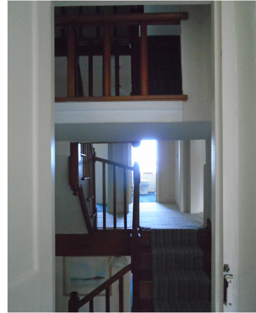
Figure 18 - View to first floor landing with half landing to the attic above
