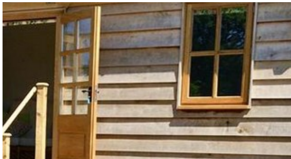
Example of natural wood finish to external windows and doors
