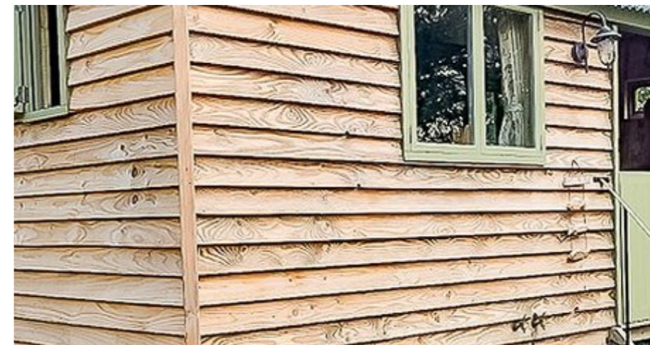
Example of pastel shade painting of external timbers and doors
